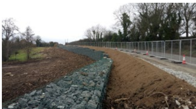
Stabilisation works at Grange Nenagh R493 Nenagh to Puckane road
