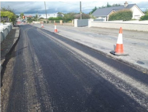
Temporary roadworks carried out on the N62 Templemore
