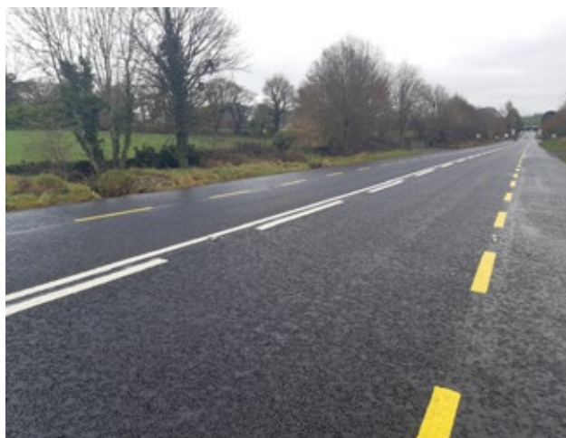
Completed works on the R445 Nenagh to Toomevara Road.
