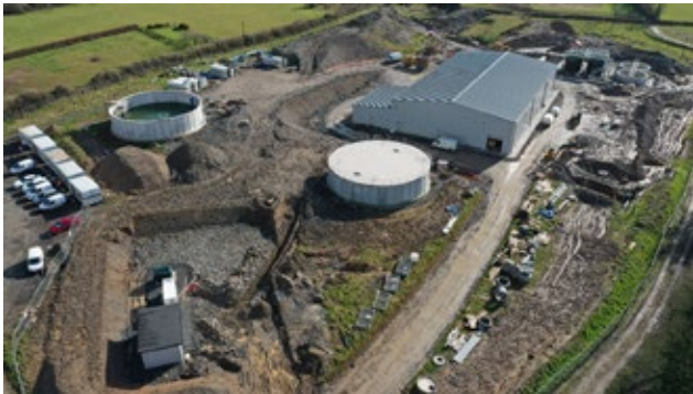
Thurles Water Treatment Plant
