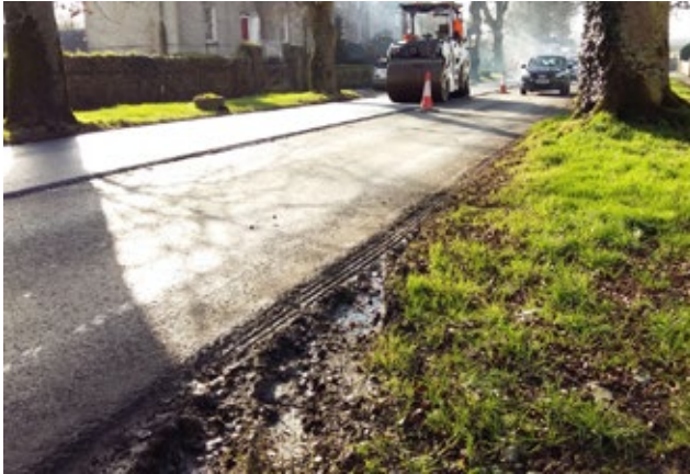
Road surfacing works - N52 Borrisokane Street Improvement Works
