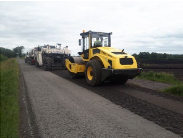
Road recycling works carried out at Knock, Roscrea
