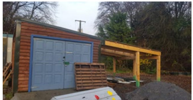
Extension to a men's sheds funded under the CEP.
