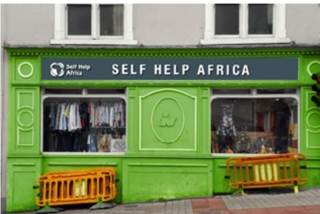
No. 17-19 Main Street, Tipperary - before and after works
