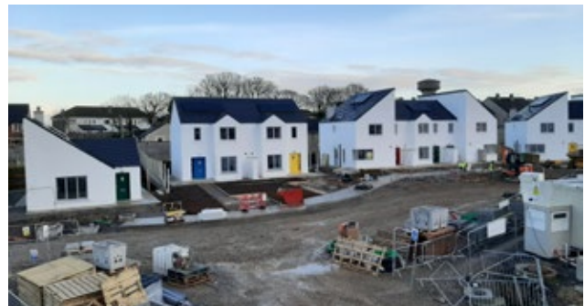
Glencoonor Housing Scheme Clonmel Under Construction – 26 units
