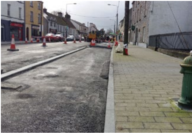
Road surfacing works - N52 Borrisokane Street Improvement Works
