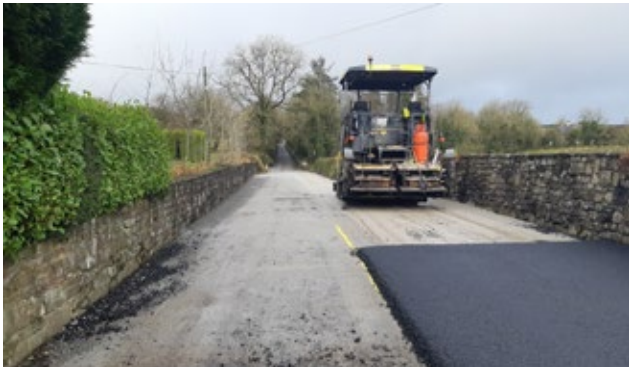
Roadworks in Progress in Killoscully
