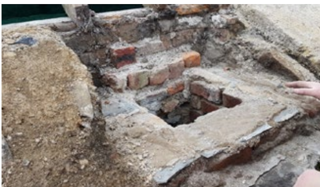
Cutting out of cement mortar by hand
