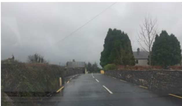
Completed works in Killoscully
