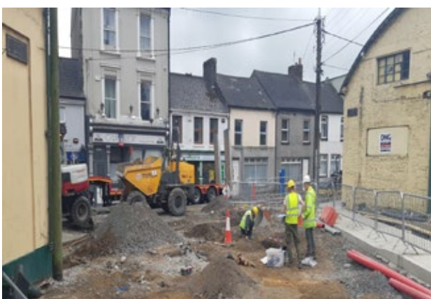
N24 Davitt Street/Church Street, Tipperary Town
