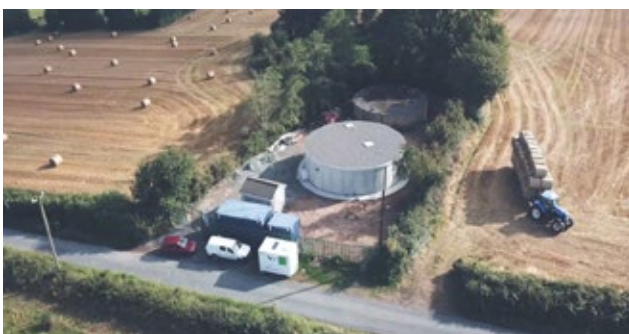
Ardfinnan Regional Water Supply Scheme - Kilroe Reservoir
