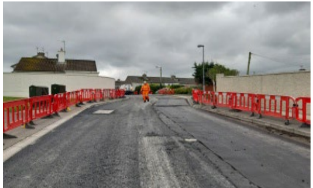
Canon Hayes resurfacing works
