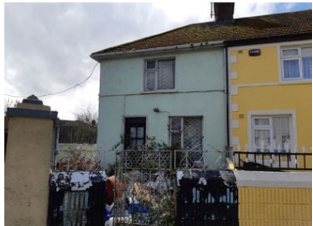
14 St Michaels Avenue, Tipperary Town. - Currently undergoing renovation. As part of the works the house will get new Windows and external insulation.
