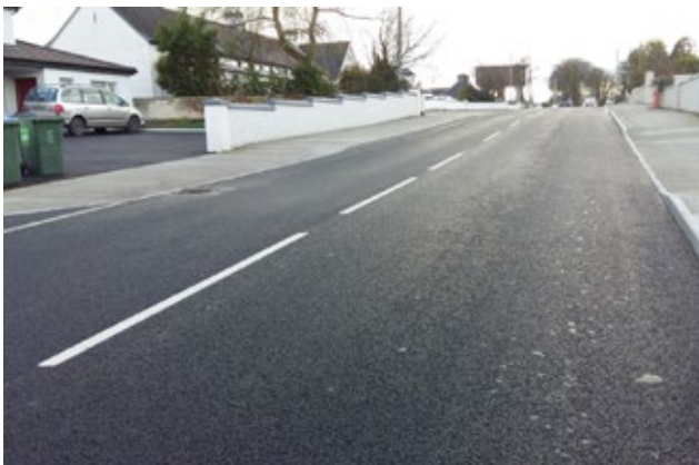
Completed footpaths and pavement works near Borrisokane Primary School
