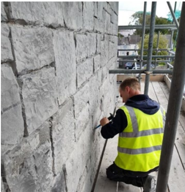
Cutting out of cement mortar by hand
