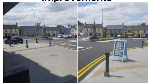
Lower Gate in Cashel improvements
