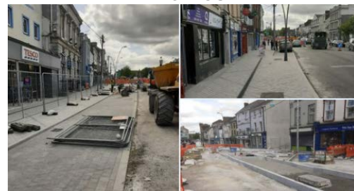
Work in progress Liberty Square Thurles
