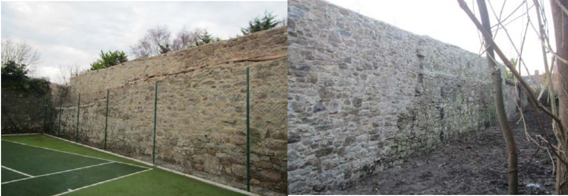
Figure 1: Works complete at Carrick on Suir
