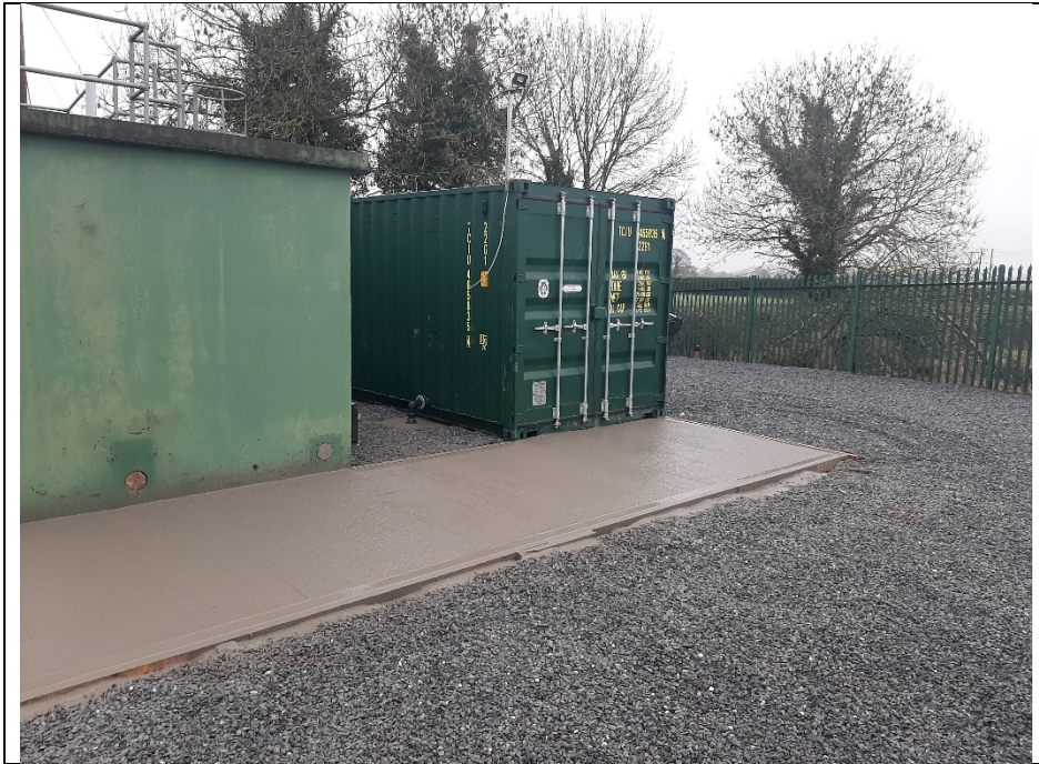
Dualla Public Water Supply
