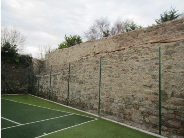
Figure 1: Works complete at Carrick on Suir
