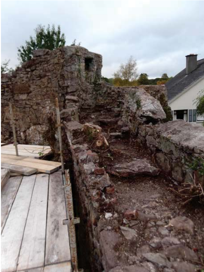
Top of Wall Walk at Carrick on Suir
