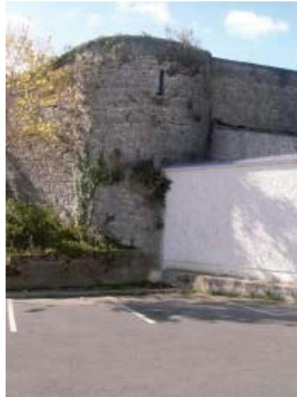
Corner tower Fethard
