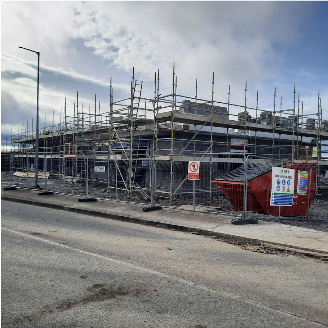
New Cashel Fire Station
