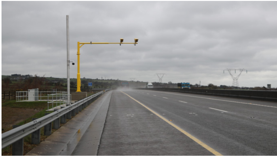
Figure 3: Image of Ireland’s 1st Mainline Motorway Average Speed Camera System on the M7 between Junction 26, Nenagh and Junction 27, Birdhill.
