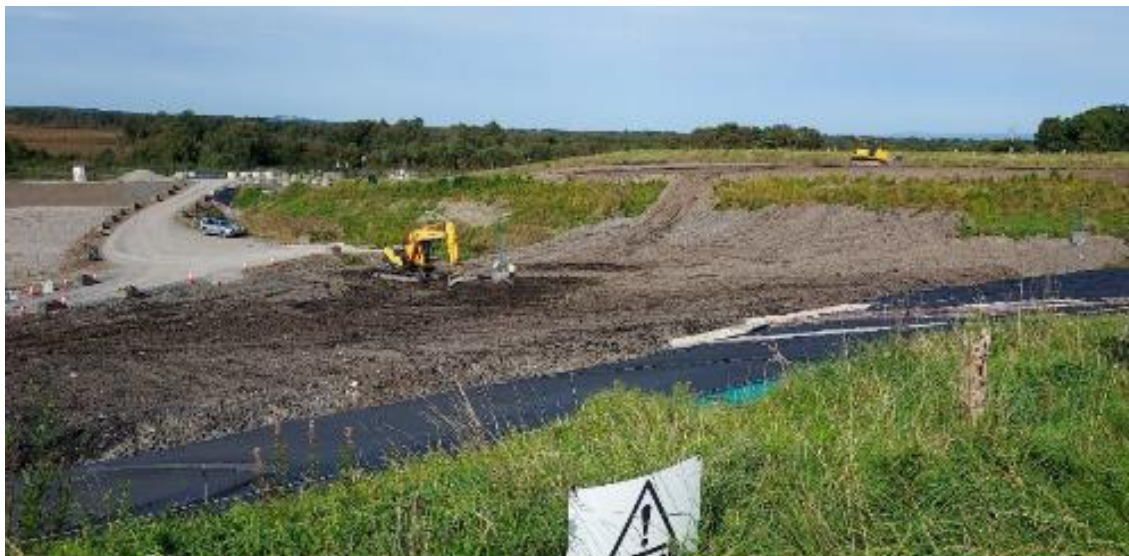
Ballaghveny landfill-Cell 10b being filled with waste, 05th September 2023
