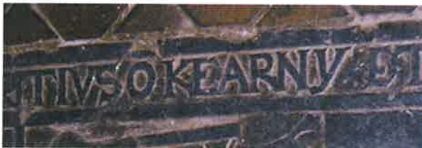
False Relief – where the letters of the memorial have been carved into the surface of the memorial to give the impression that the letters are in relief but they are still flush with the surface of the memorial Relief – where the letters are raised above the surface of the memorial
