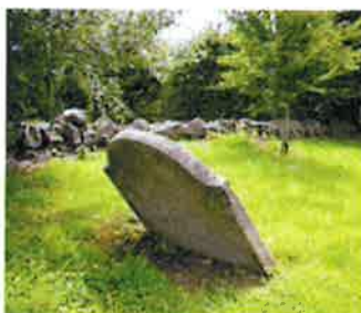
This well preserved inscription is protected from weathering due to its leaning position. This memorial should not be re-erected into an upright position as this would lead to the weathering of the inscription and also detract from the character of the graveyard.
