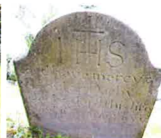
This well preserved inscription is protected from weathering due to its leaning position. This memorial should not be re-erected into an upright position as this would lead to the weathering of the inscription and also detract from the character of the graveyard.
