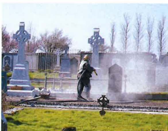
The sandblasting of memorials speeds up the process of decay of stone and should be avoided
