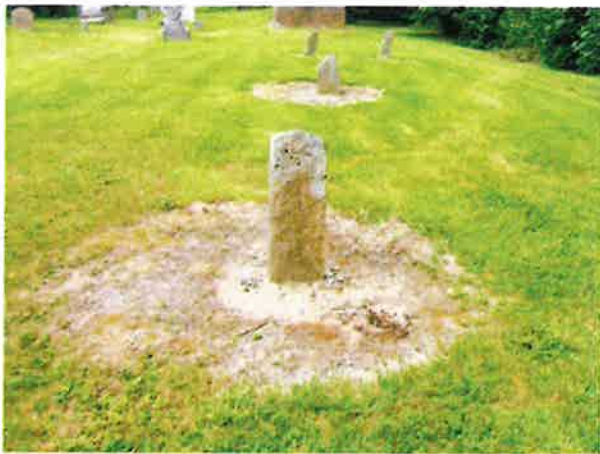
Sod has been removed from the base of this memorial which will allow weeds and ivy to become established
