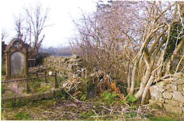
The planting of trees near graveyard walls should be avoided as their root system will eventually cause collapse, as shown here at Antrim, Co. Laois. There is a need to monitor self seeding trees in a graveyard and remove saplings near walls to avoid future long term damage and costs
