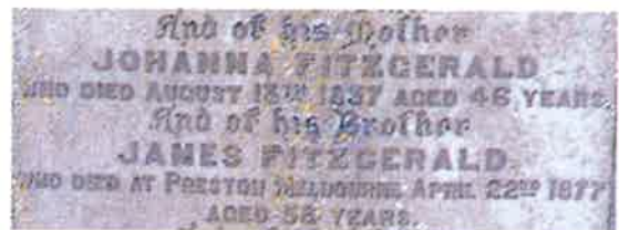
Applied – where the letters are attached onto the surface (appliqué) of the memorials.
