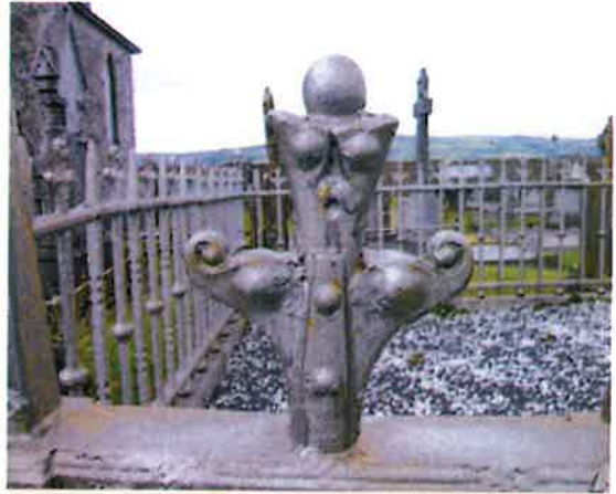
St Augustines graveyard, Co. Waterford, iron railings (1879 AD)
