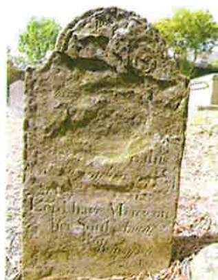
Birr, Co. Offaly, memorial inscription has been lost due to natural weathering process
