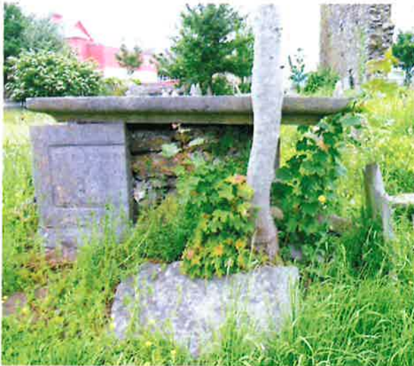
The damage caused by a Sycamore tree can be clearly seen in this graveyard
