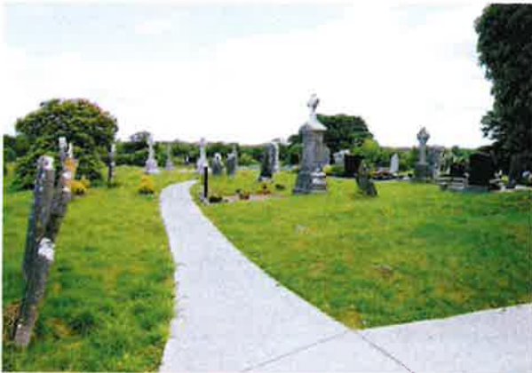
A concrete pathway can have a negative effect on graveyard character and has long term maintenance and health and safety issues
