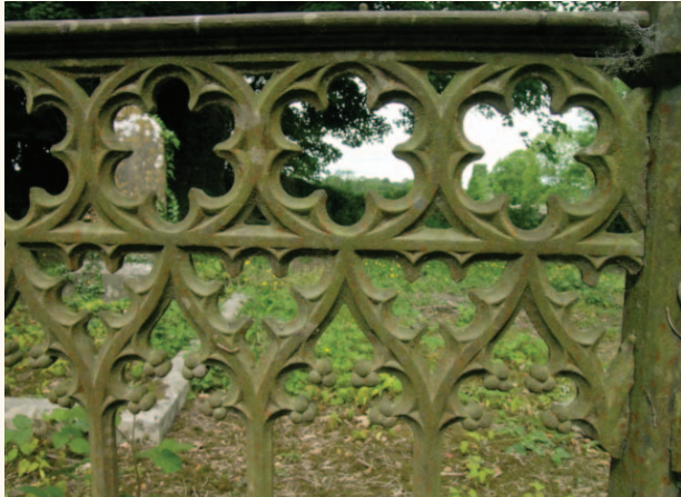
Cast iron memorial railings in Whitechurch, Co. Waterford
