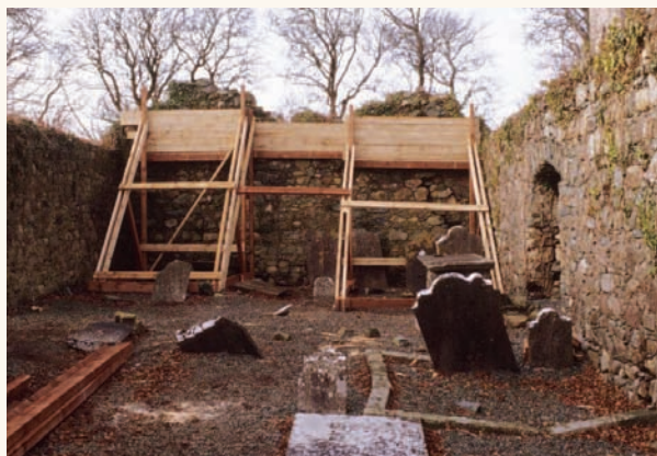
Ongoing conservation works with timber bracing used to support a masonry wall temporarily at Stradbally, Co. Waterford
