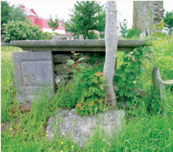
The damage caused by a Sycamore tree can be clearly seen in this graveyard
