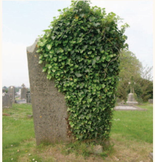
Weedkiller has been sprayed around the base of this headstone allowing the ivy to thrive
