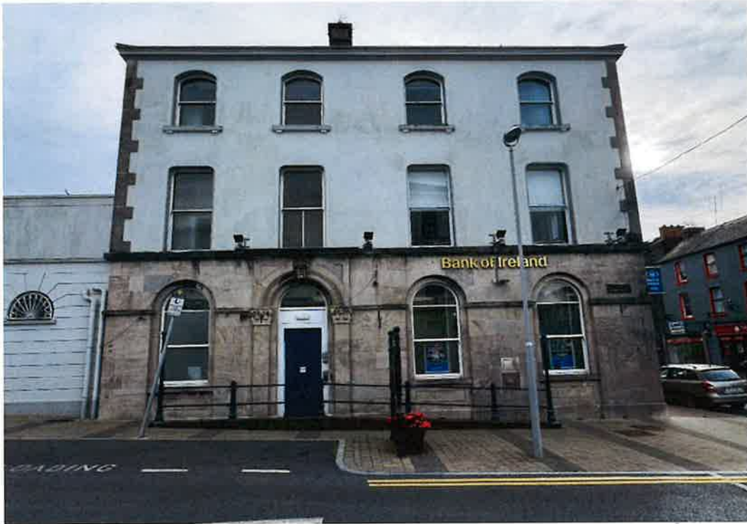
Plate 3: Market Place (western) elevation of the protected structure
