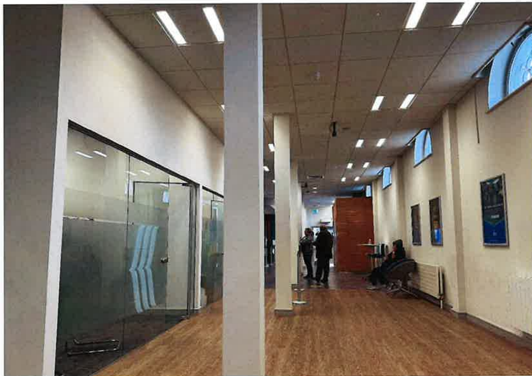
Plate 7: View of interior of the rear return of the banking hall – the area is entirely modern and is devoid of fabric of architectural heritage significance.
