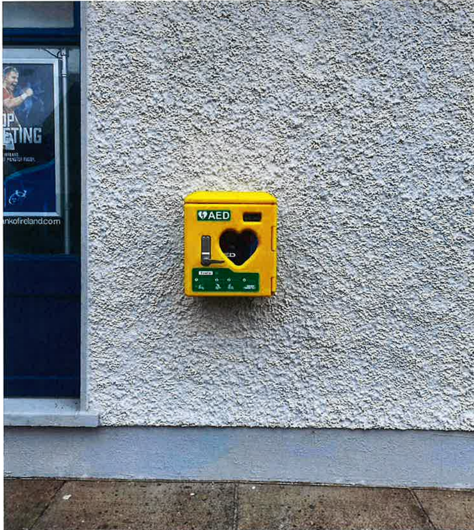
Plate 9: Example of the defibrillator to be installed
