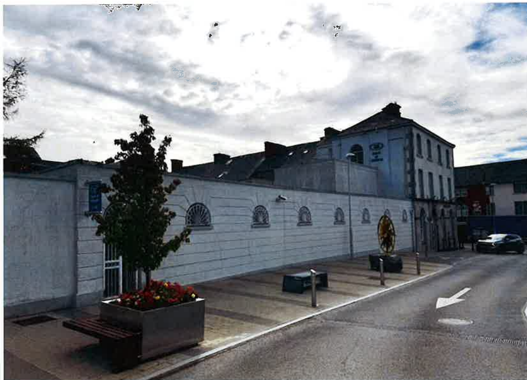
Plate 4: Eight-bay banking hall extension that presents to Market Place. This is a late twentieth-century addition.
