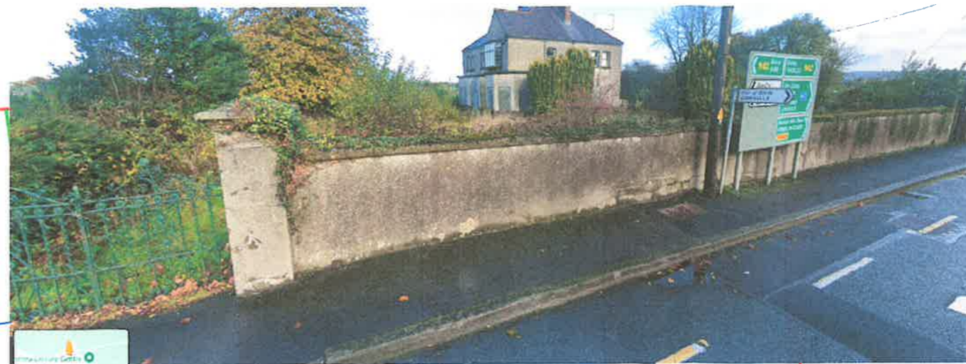
Existing Entrance Wall & Pillars
