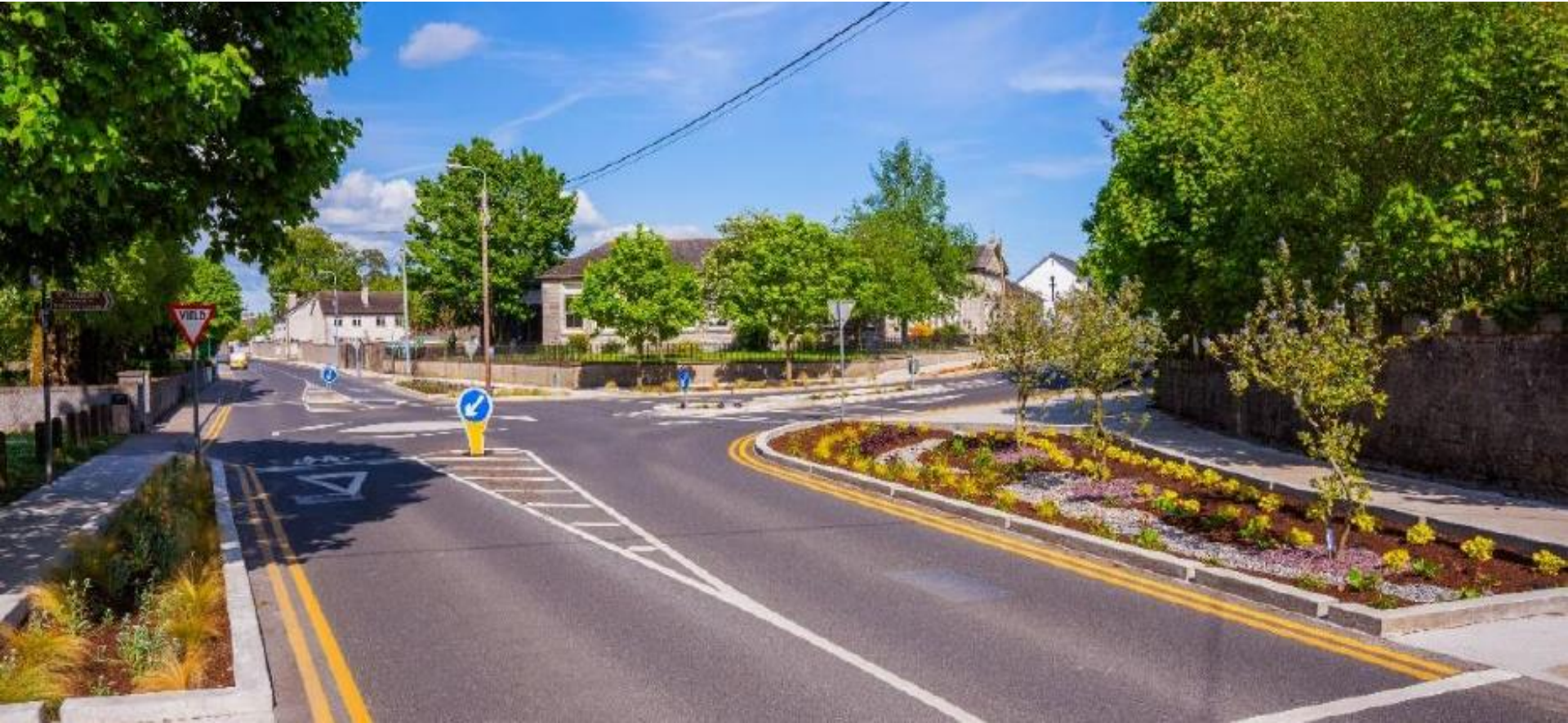
Completed Rain Garden Project (Bioretention Areas)
