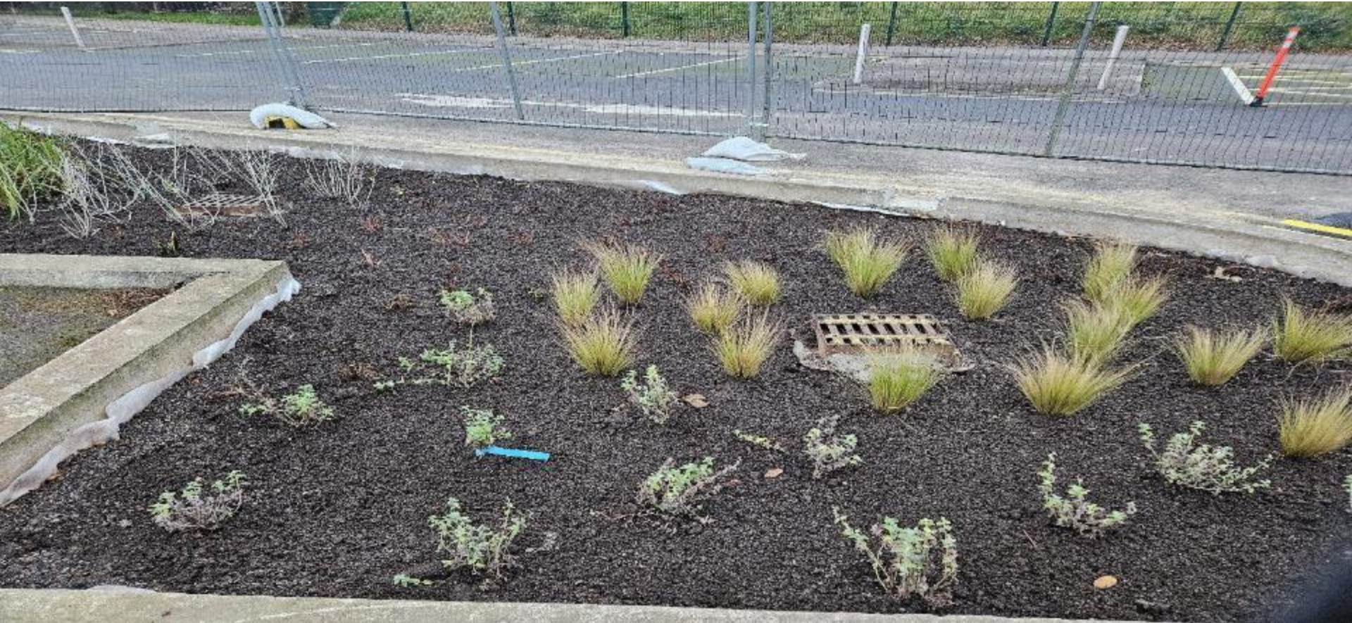
Bioretention Areas (Rain Gardens) – Clonmel (engineer Eamonn O’Connell)
