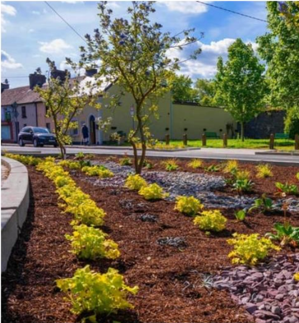
Carlow's rain gardens are a free draining soil mix that cleans, stores and conveys runoff water
