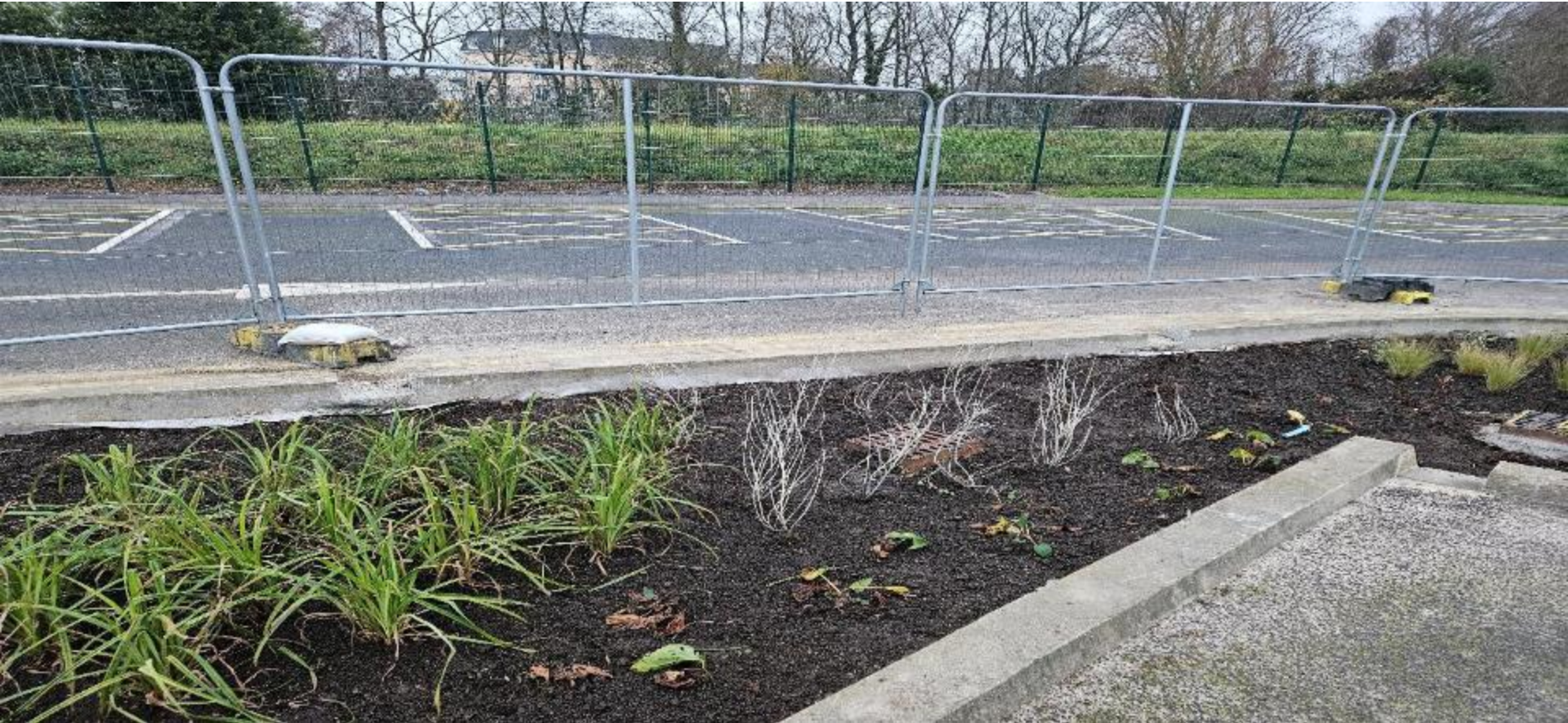
Bioretention Areas (Rain Gardens) – Clonmel
