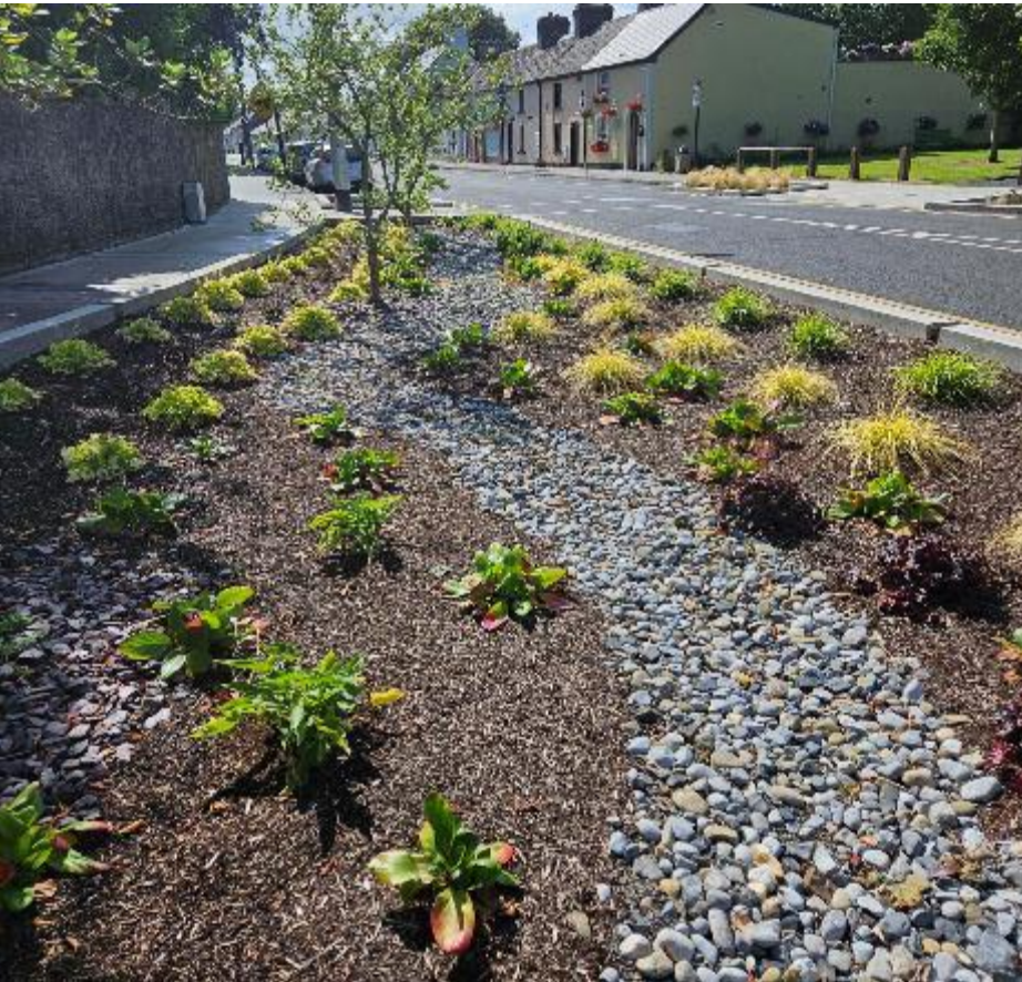
Completed Rain Garden Project (Bioretention Areas)
