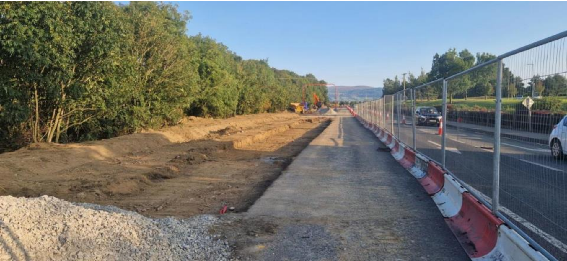
Bioretention Areas (Rain Gardens) – Clonmel (engineer – Gillian Flynn)
