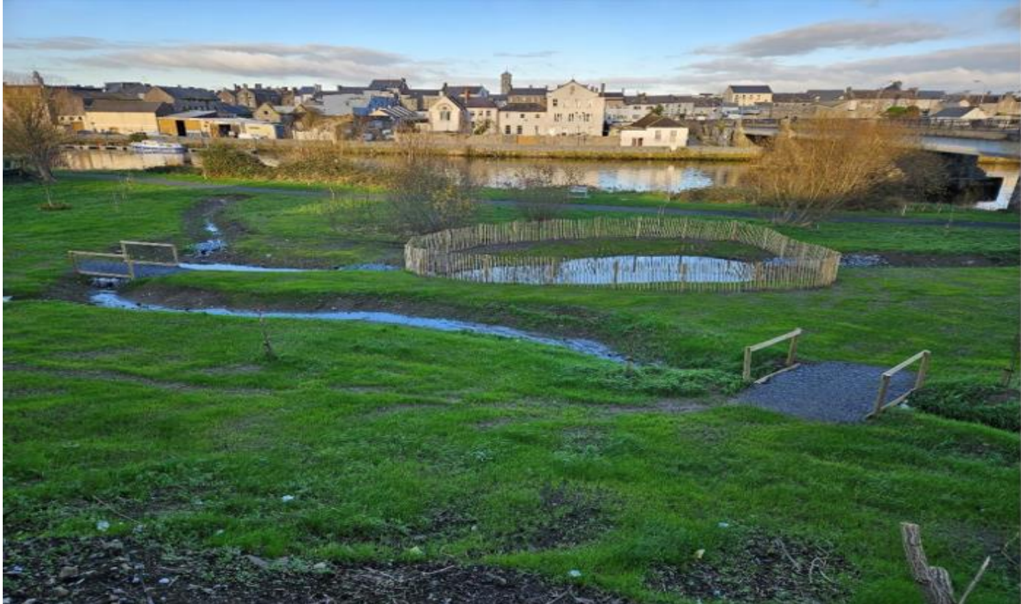
NbS features (swales & interception ponds) – The Bog Field, Carrick-on-Suir
