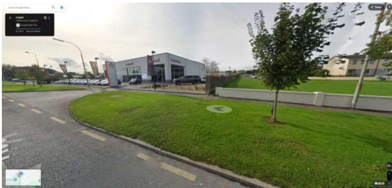
Figure 2 Subject Site (Google Street View 2019)
