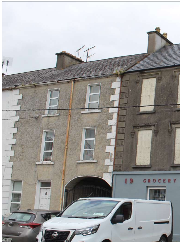
Figure 1: South-east elevation of subject building in June 2024
