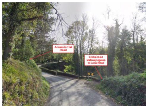
Figure 18: View on Road from Embanked Egress to Bridge
