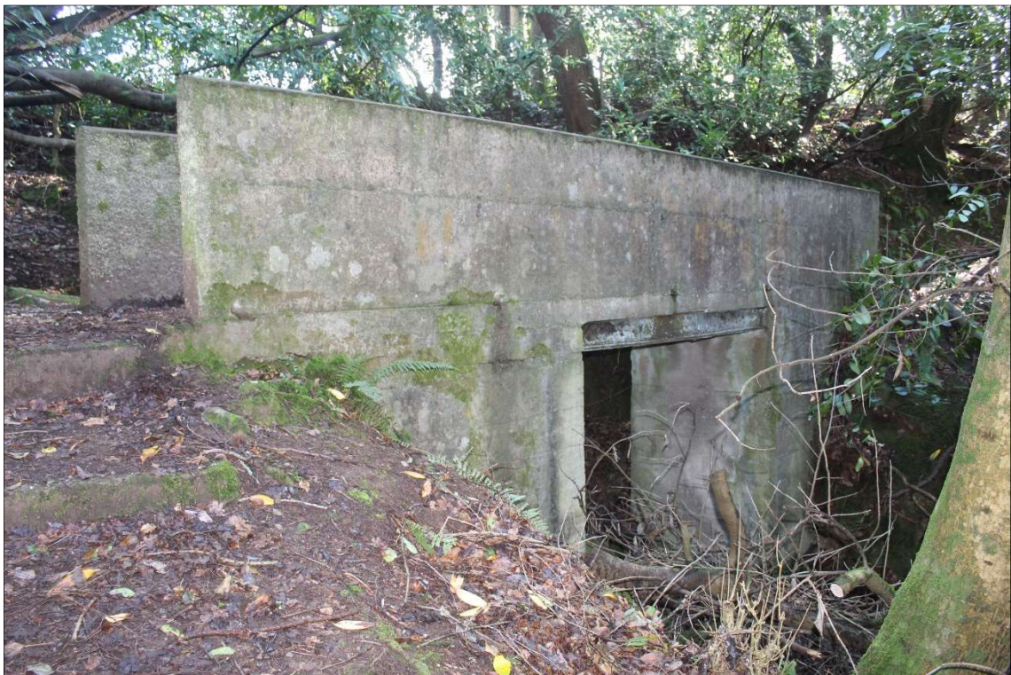
Figure 11: South-west elevation of replacement concrete bridge over streambed of tributary to Clare River, approximately 475m east of Clare Bridge. Proposed replacement of this structure to provide improved access at this point (the historic location of a previous foot bridge) will not result in any loss of historic fabric and will be appropriate to retain a pedestrian way along this historic route.
