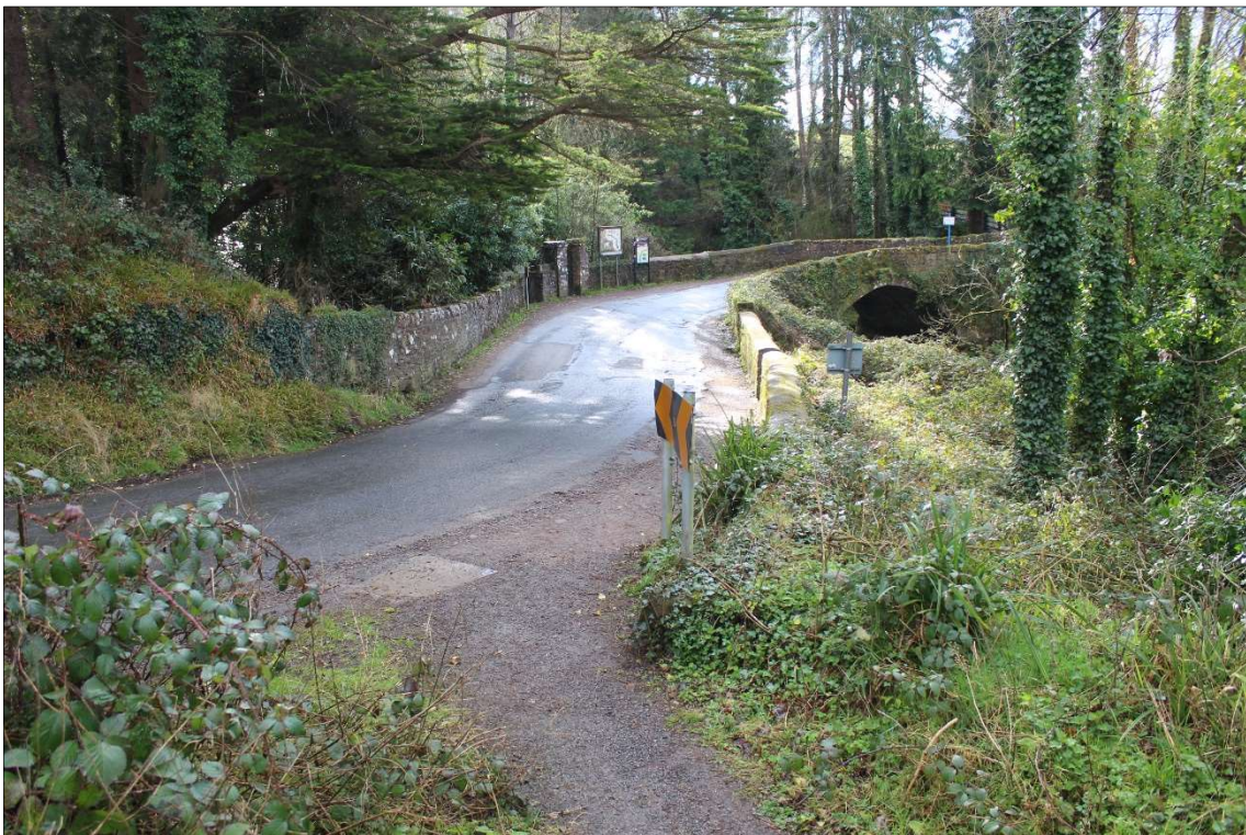
Figure 7: Upstream, west elevation of Clare Bridge from existing footpath installed behind historic roadside boundary in recent years. Proposed works to upgrade Clare Glens walk will have no impact on existing views to or from Clare Bridge.
