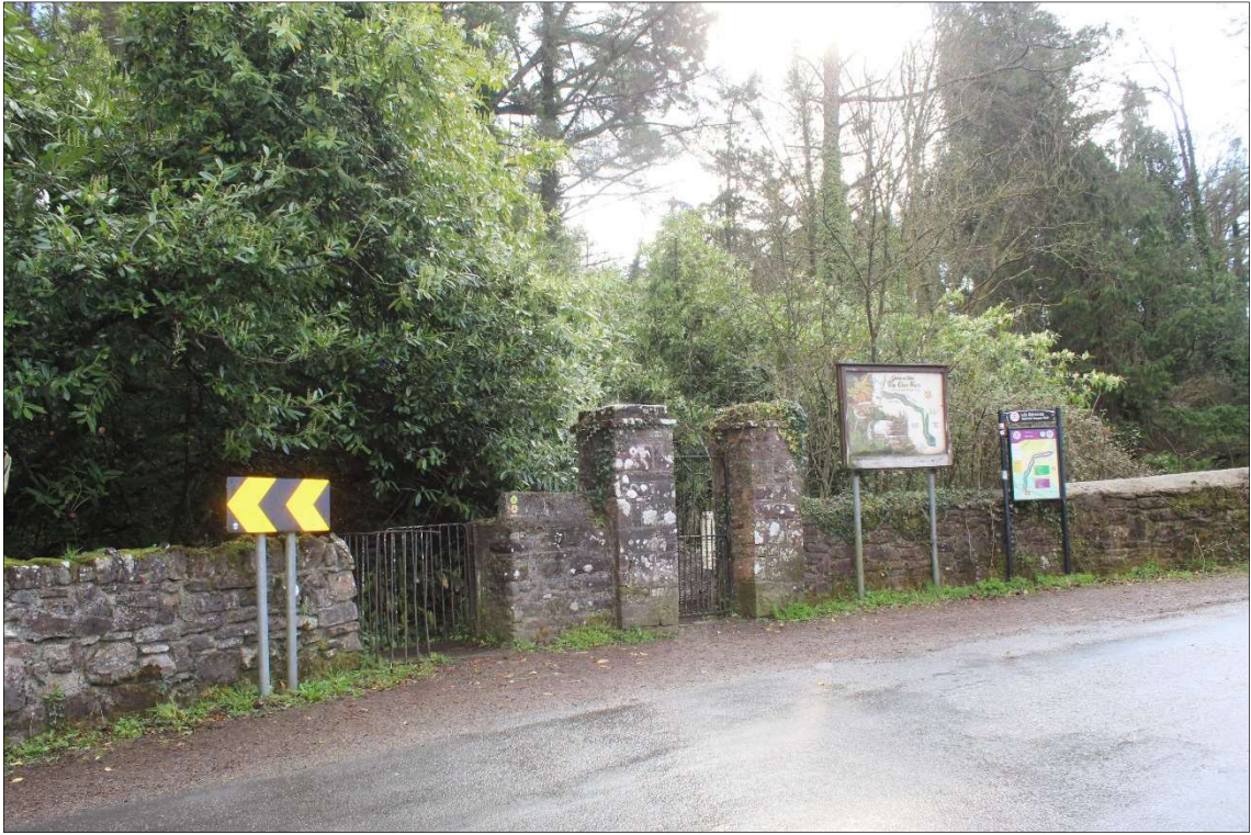
Figure 8: Existing historic gateway (and later kissing gate) immediately north of Clare Bridge on downstream (east) approach wall with wrought-iron gate on rubble sandstone piers.
