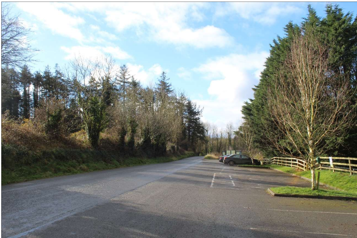
Figure 3: View to south along L-2164-0 with 51m of existing roadside boundary proposed to be removed to facilitate sight-lines for new vehicular and pedestrian entrance to walkway with similar stone and earth embankment with native hedgerow species to be reinstated as roadside boundary to both sides of proposed new timber entrance gates.
