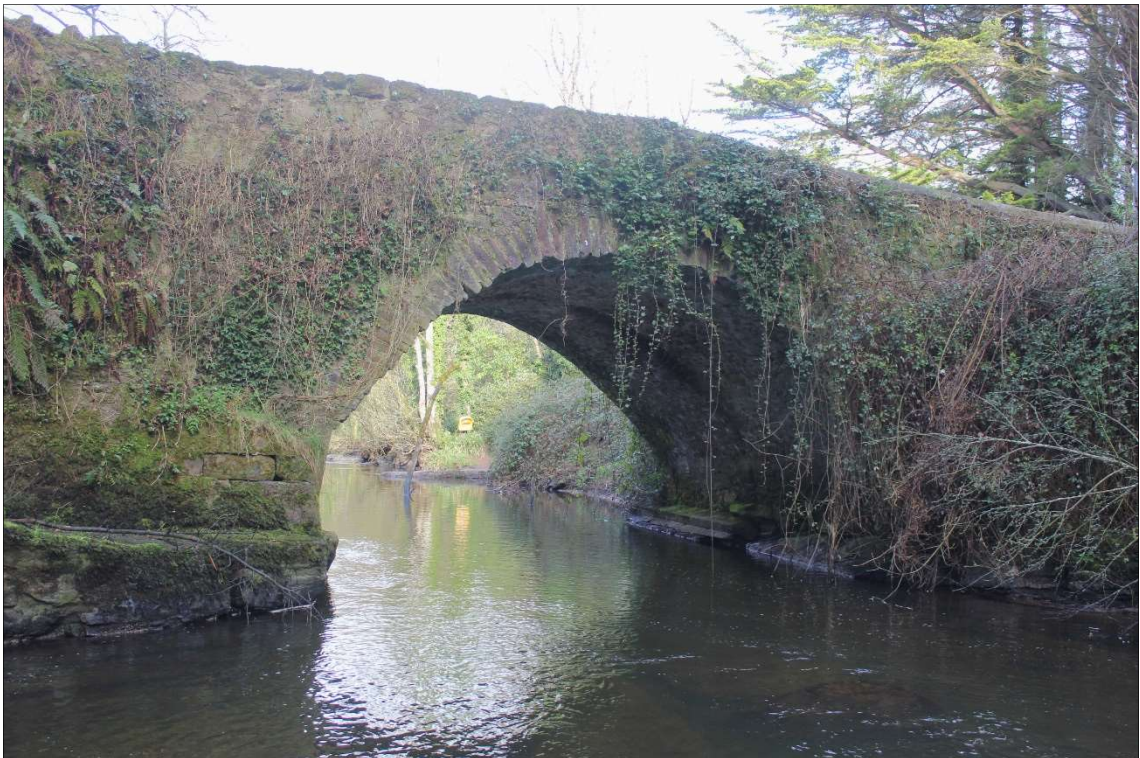
Figure 9: Downstream, east elevation of Clare Bridge from southern bank of Clare River.
