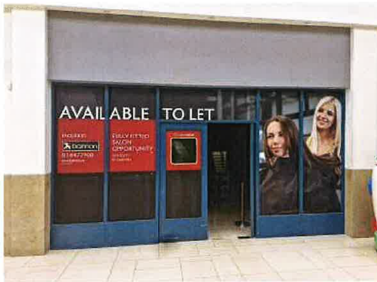
Front of existing Hair Salon. The doors are to be removed and a shutter door system installed to match the existing Paul Byron Shoe Shop
