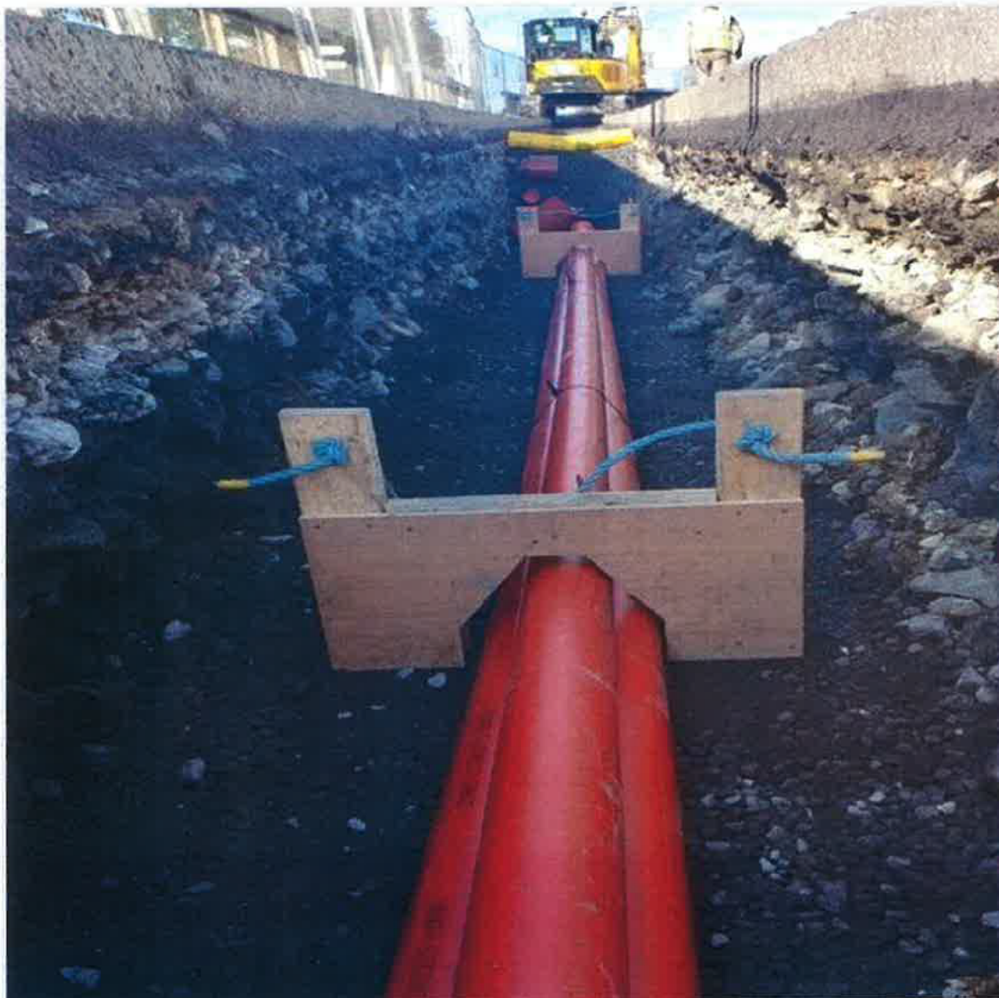
Figure 2: Typical underground duct installation
