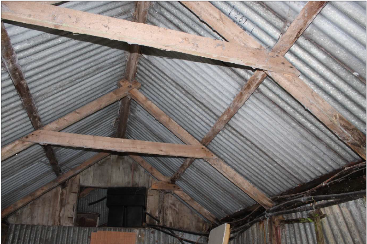
Figure 4: Detail of simple internal roof structure within existing shed, all of which re-useable timber and corrugated steel will be salvaged and reused following appropriate, localised repairs.
