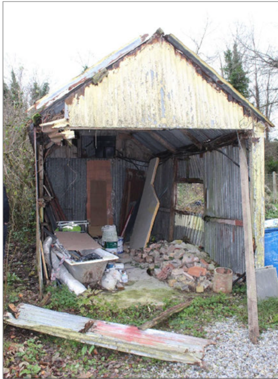
Figure 2: North-west open gable end of subject shed proposed to be closed with corrugated steel-clad doors with salvaged, decorative bargeboard repaired and reinstated to this elevation.
