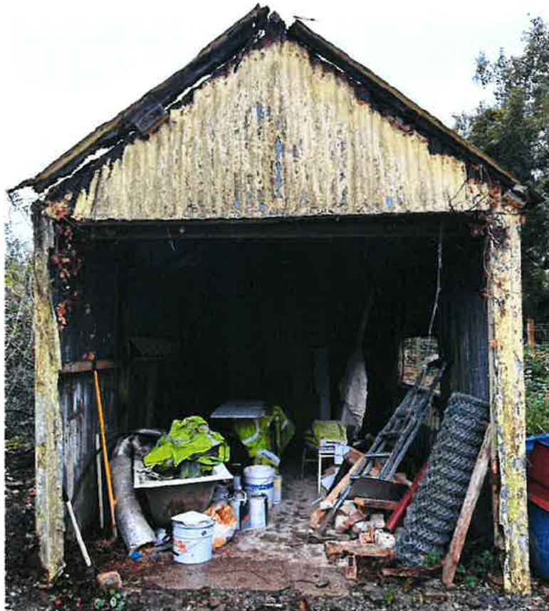
Figure 9: Timber-framed garage clad in corrugated-iron situ
