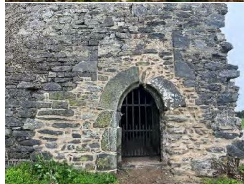
Before and after pictures of the east door at Loughloher Castle
