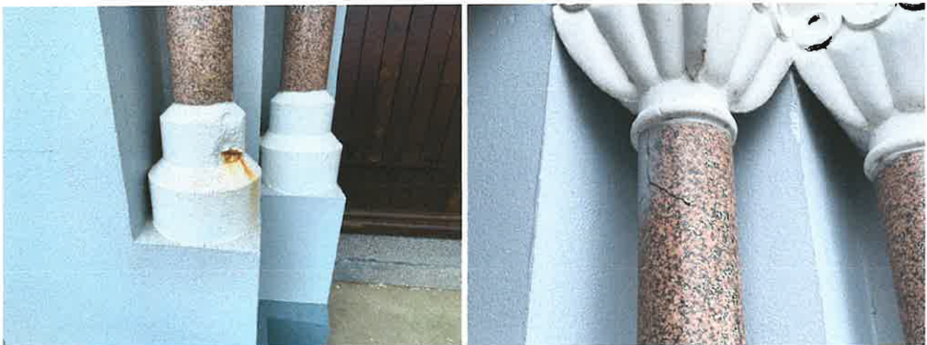
Photo 13; North side of entrance porch column, there is evidence of rusting to the base of the column, due to loss of concrete cover resulting in steel reinforcing rusting. Photo 14; Fracture in marble column at north side of entrance porch.
