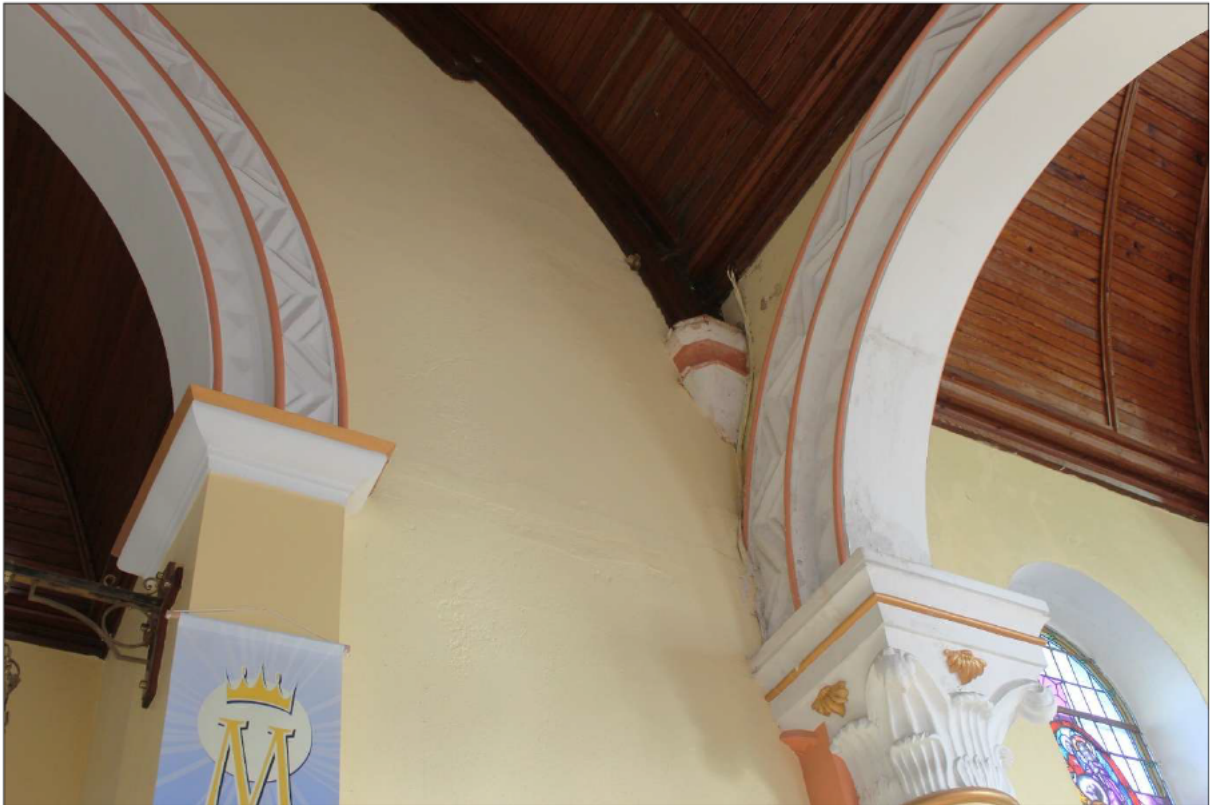
Figure 7: Moisture damage evident to painted plaster wall surfaces beneath base of defective lead valley on east side of south transept. Damaged internal surfaces to be made good using appropriate materials and surface finish to match existing.
