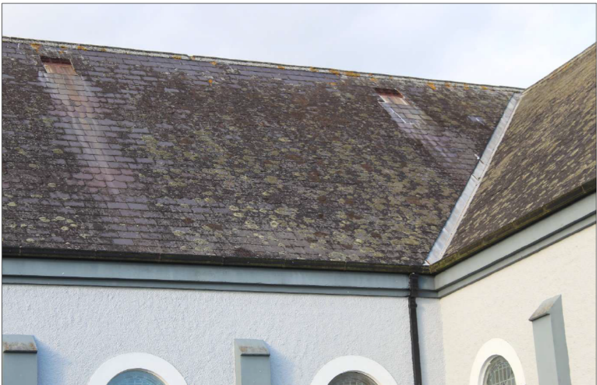
Figure 4: Existing roof valley on west side of south transept. Valley to be re-lined and slates to be re-fixed to match existing
