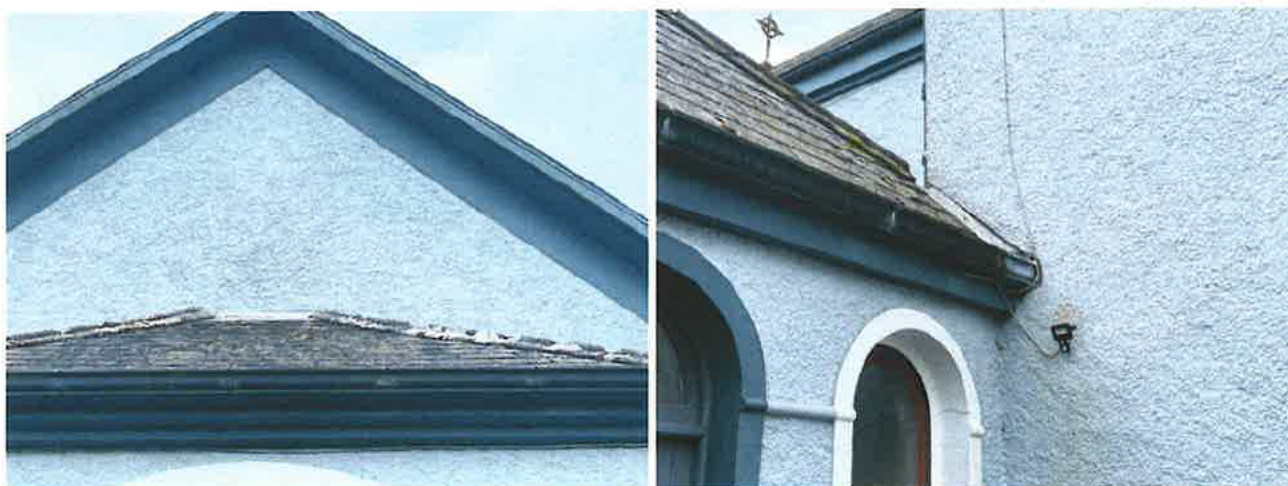
Photo 19; There is a significant crack to the gable wall over the apse roof on the west wall. Photo 20; There is evidence of water overflowing / leaking from the sacristy roof flashing / gutter onto the east wall of the apse.
