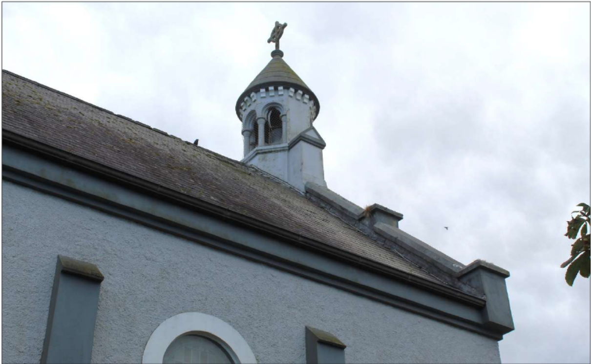
Figure 3: Lead abutment flashing to inside of west parapet and around base of bellcote to be inspected and repaired locally where necessary. Lower courses of slate on this north elevation of nave to be removed, repairs to timber roof structure carried out where necessary and natural slate to be reinstated. Existing extruded aluminium gutter here to be replaced with more durable cast aluminium
