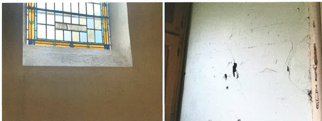
Photo 33; Evidence of water ingress to window on north wall of nave, adjacent to location of rainwater downpipe externally. Photo 34; Damage to lath & plaster wall in sacristy store.
