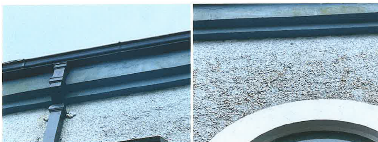
Photo 23; Evidence of potentially bulging plaster over window head on north wall of nave. Photo 24; Evidence of previous repairs to render above window, north wall of nave.
