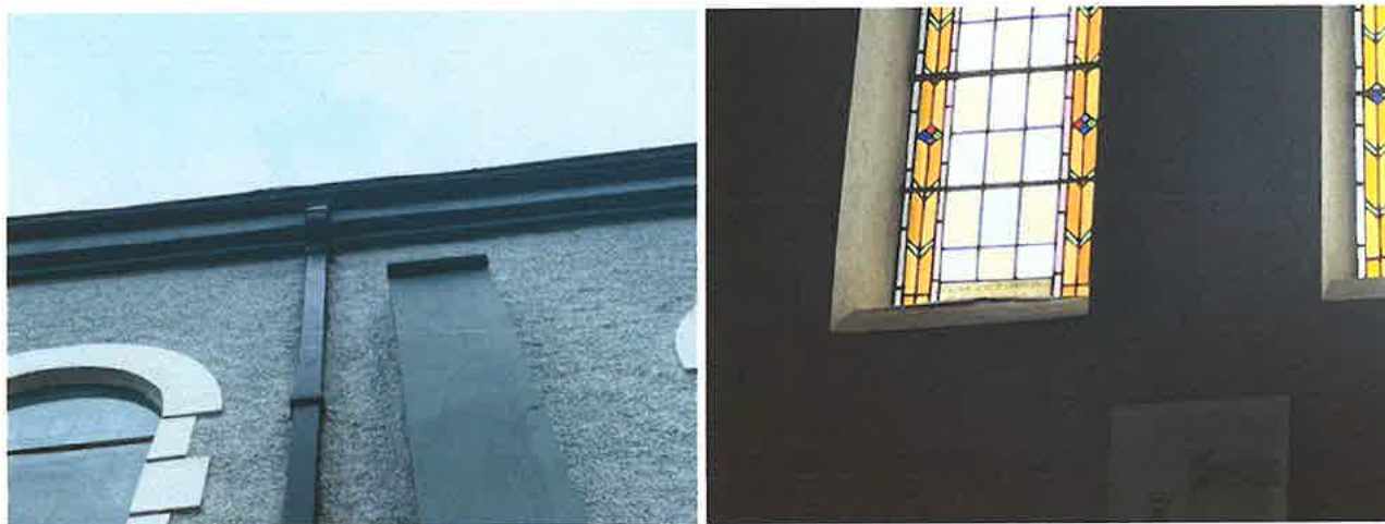
Photo 38; Rainwater downpipe causing staining / water ingress, between window W.04 & 05. Photo 39; Interior damage to be cleaned down and reinstated.
