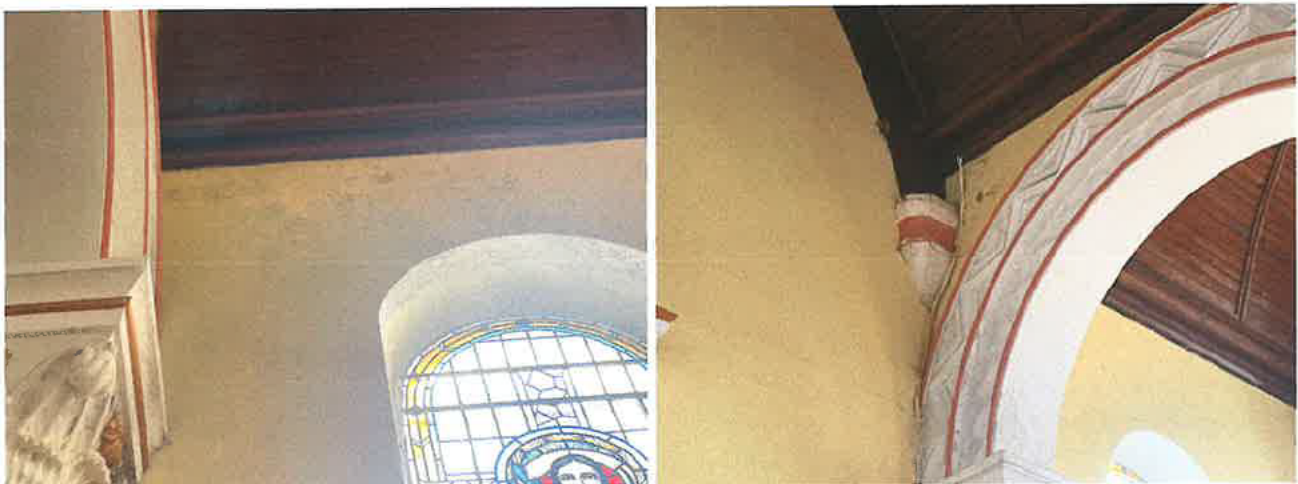
Photo 29; Evidence of water ingress to east wall of south transept, near roof valley. Photo 30; Evidence of water ingress to east wall of apse, near roof valley.
