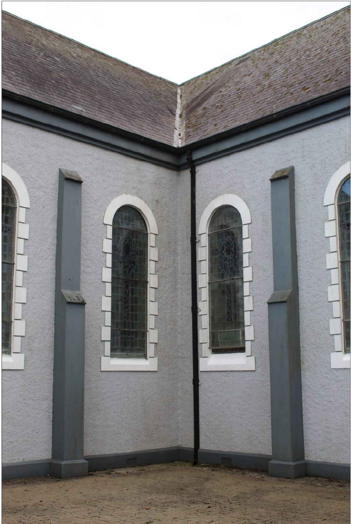
Figure 2: Existing roof valley on west side of north transept. Valley to be re-lined, lower courses of slates on both elevations shown in photograph above to be repaired, gutters to north elevation of nave (right side of photograph) to be replaced, rainwater gulley beneath existing downpipes to be cleaned and inspected for damage.
