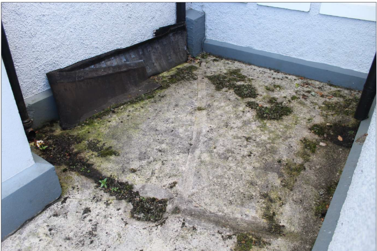
Figure 6: Existing concrete ground surface to be removed from between south transept and sacristy with new stormwater gulleys to be installed directly beneath downpipes
