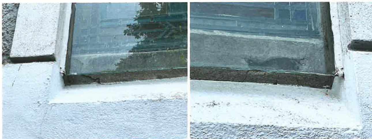
Photo 21 & 22; Damage to concrete cill to window, perhaps due to metal tie-bars in concrete rusting and resulting on the concrete spalling / cracking.
