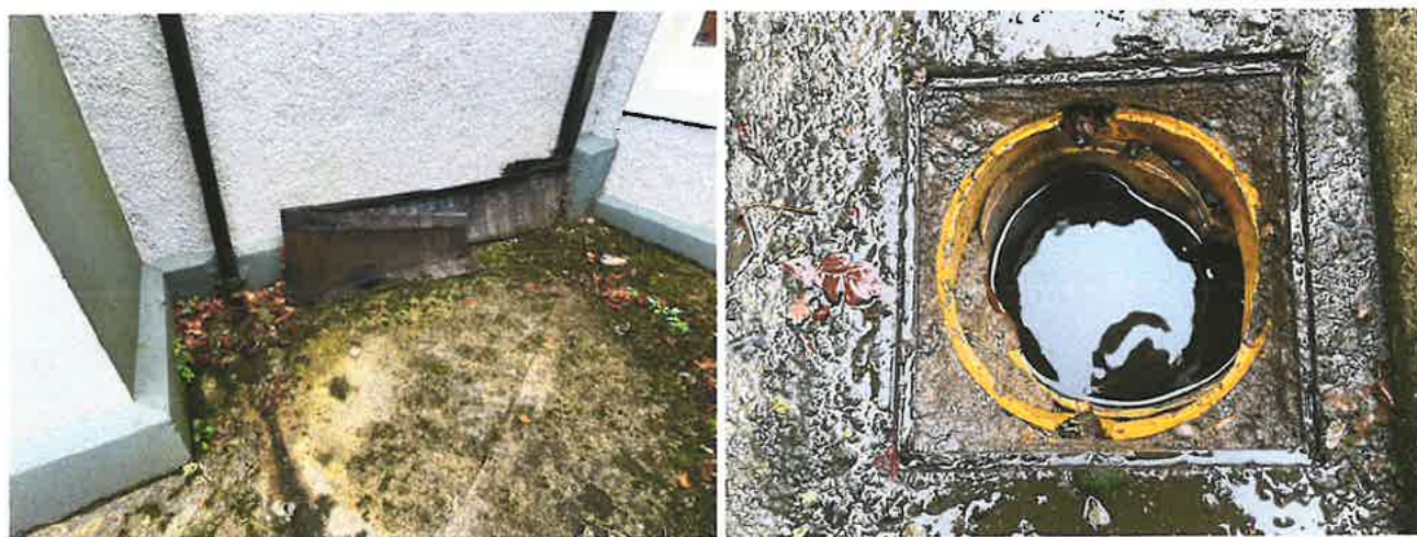
Photo 37; Existing concrete slab to be removed to investigate subsoil drainage, and replaced with permeable surface.
