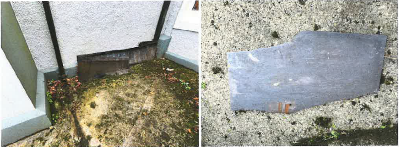
Photo 27; The area to the east of the sacristy and the south transept has three rainwater pipes discharging onto a concrete slab, with limited subsoil drainage. Photo 28; This roof slate has fallen from the west face of the south transept roof, it will have been damaged by falling, however the slate has been significantly weathered over time, with the nail holes weakened. This could be indicative of what may be expected if the entire roof was to be re-slatted, with considerable slate replacement required.
