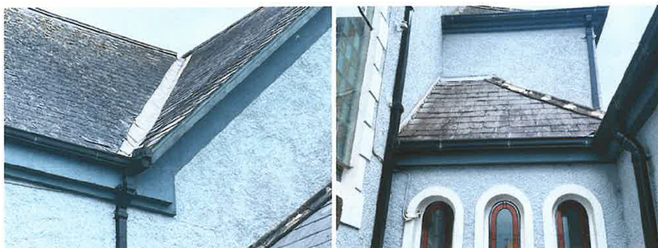
Photo 25; The roof valley linings to the east facing pitch of south transept and nave roof appears to have been replaced, and that a gutter stop has been installed, perhaps to limit the rainwater flow, due to the gutter overflowing.. Photo 26; Evidence of previous repairs to south roof of sacristy.
