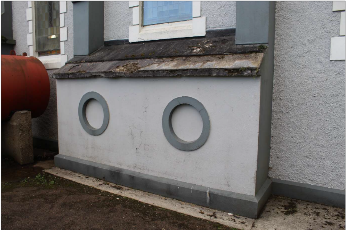
Figure 5: Existing concrete roofs to confessional outshots on east elevation to be repaired and weathered with suitable modern roof covering.
