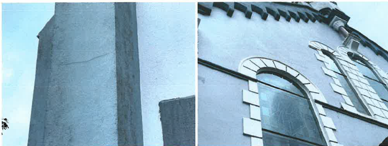
Photo 15; Cracking to render on buttress piers, these are evident throughout the building. Photo 16; There is a crack over the nave window on the west façade, which may be a source of water ingress.
