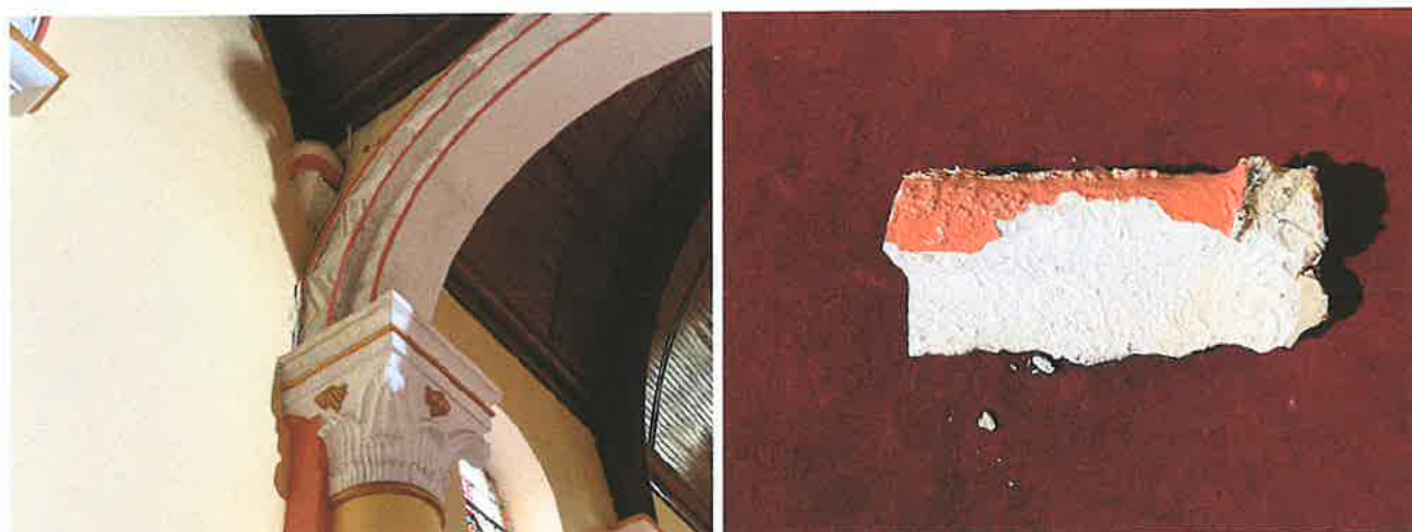
Photo 42; Damage to wall finishes. Photo 43; Damaged portion of stucco moulding.
