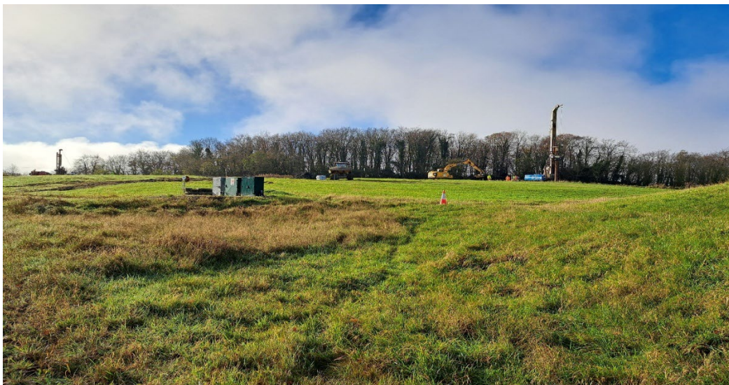
View of borehole drilling works on Cell No. 2 at Ballaghveny Landfill
