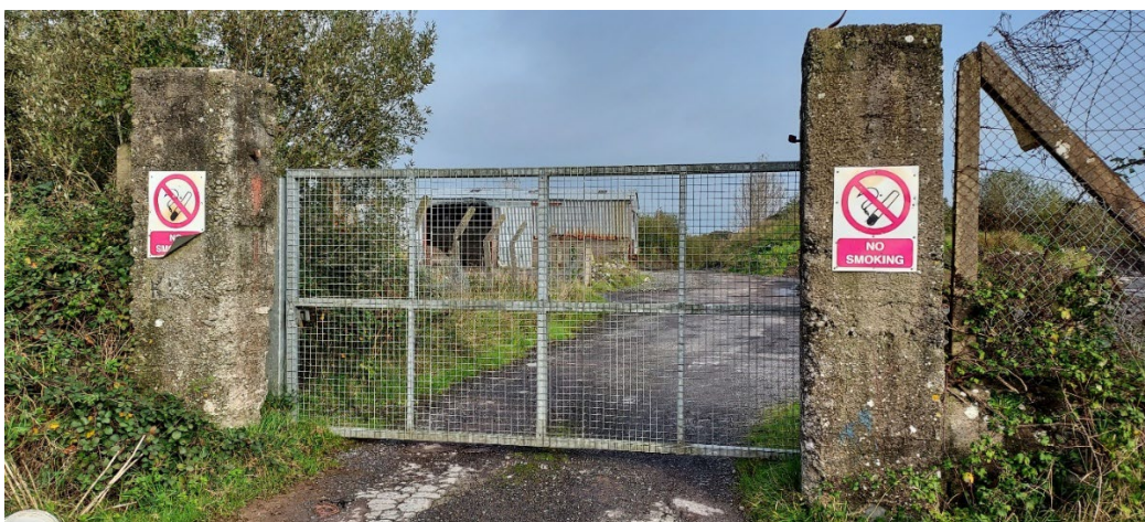
Landfill entrance gate before works commenced.
