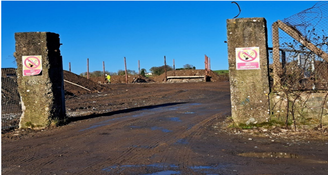
Landfill entrance gate after works commenced.
