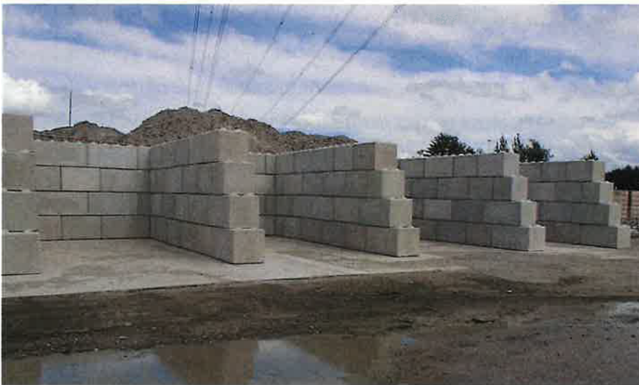
Prefabricated Concrete Block Bunkers
