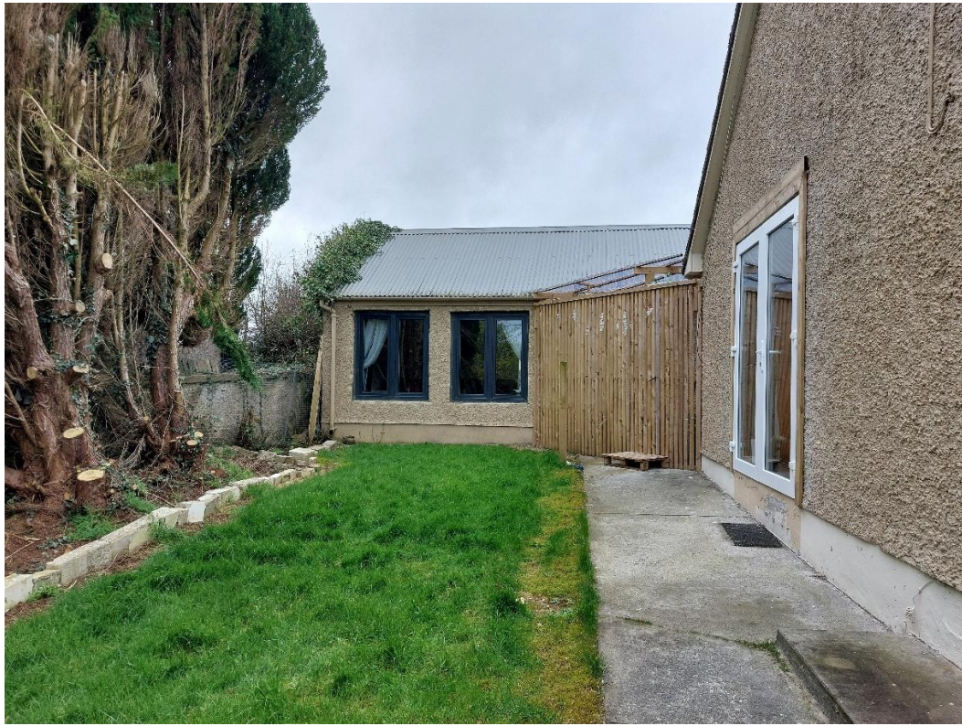
Figure 1: Windows installed to shed and door to side of dwelling
