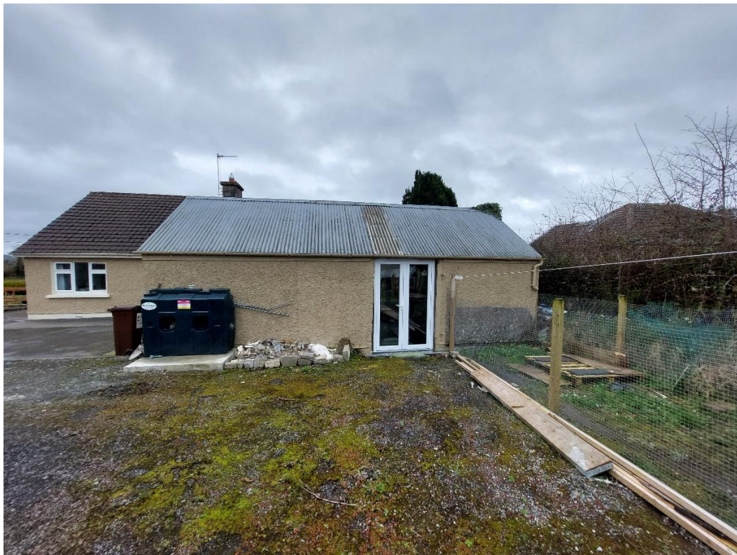
Figure 2: Door installed to garage
