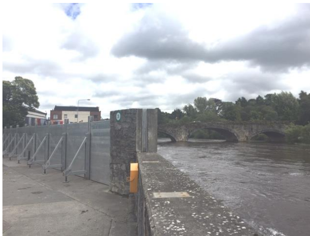
Flood Barriers in place in Clonmel
