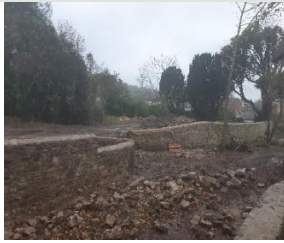
Mill Race Walls, Suir Island Repairs
