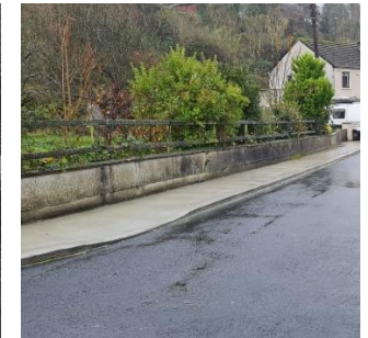
Glenegad Footpath Reinstatement
