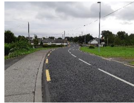
Road Resurfacing N52 Carrig Village
