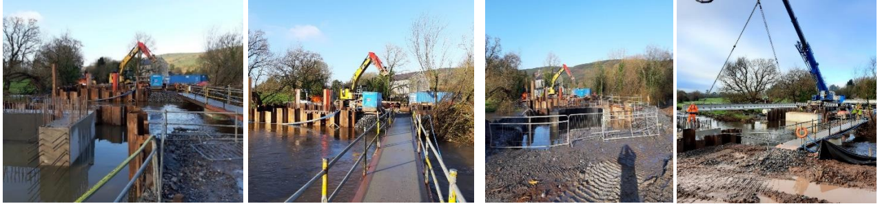
Clonbeg Bridge Works
