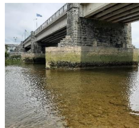
Dillon Bridge, Carrick-on-Suir
