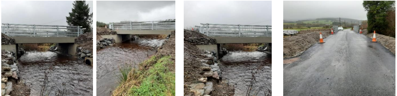
Knockshanbrittas Bridge – Reconstruction Works
