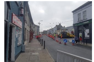
Newport R503 Main Street Works
