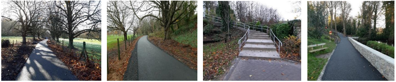
Cahir to Swiss Cottage Walkway Upgrade under ORIS Funding
