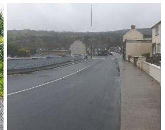
Road Resurfacing Old Bridge, Clonmel
