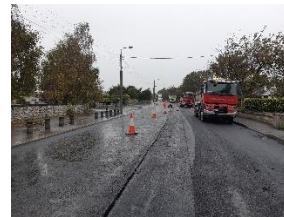
Road Resurfacing R494 Nenagh
