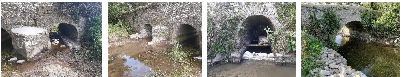
Works carried out on Bridges Coolmoyne/Ballyvadin Modeshill, Mullinahone
