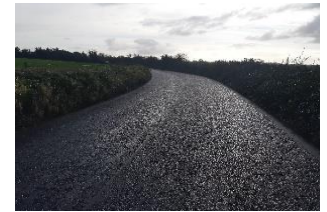
Road Resurfacing R489 Ballincor
