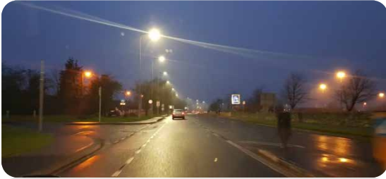
Led Public Lighting Upgrade, Nenagh
