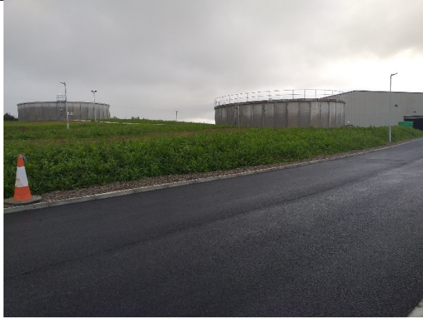
Water Treatment Plant Reservoirs
