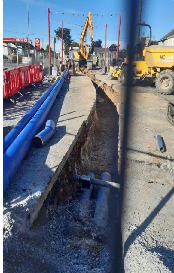
Laying of New Watermain at Abbey Road, Thurles
