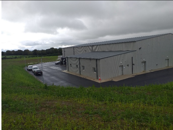
Water Treatment Plant Building
