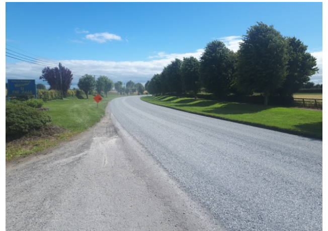
Surface dressing completed on R498 at The Ragg, Thurles
