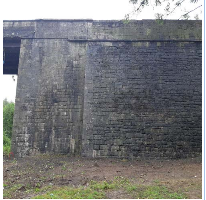
Albert Bridge Clonmel – After works
