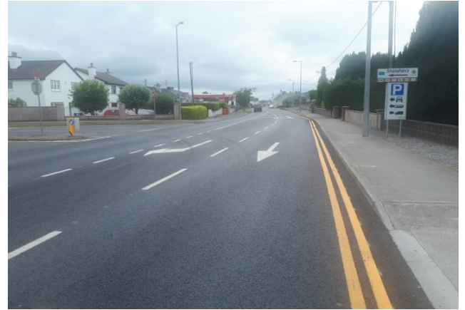
Resurfacing & relining, Main Street, Borrisoleigh
