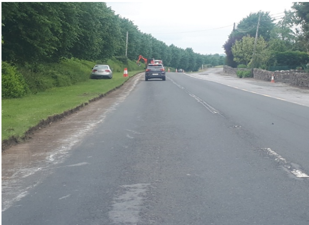
Preparation for surface dressing between The Ragg and Borrisoleigh
