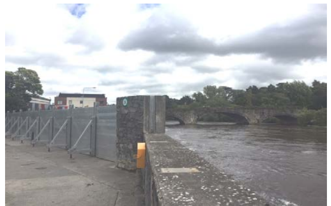
Flood Barriers in place on 25 th August in Clonmel
