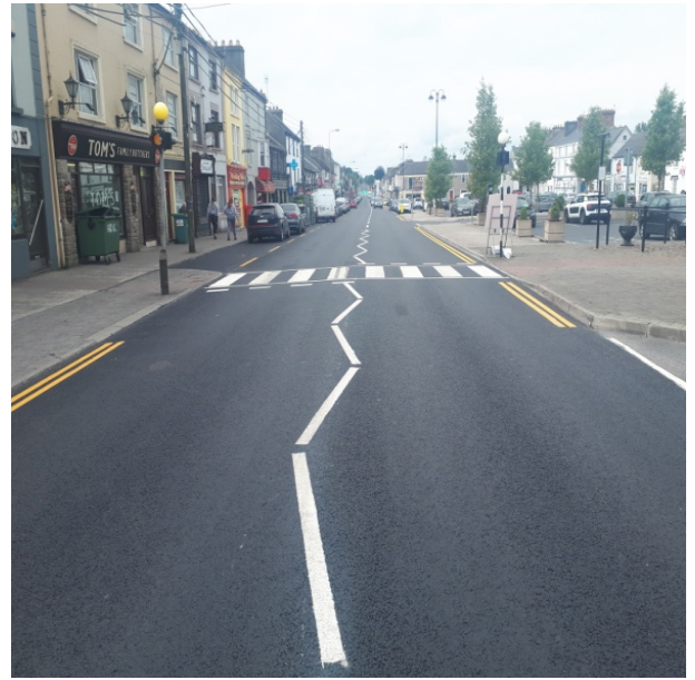
Resurfacing and relining on N62 Main Street Templemore
