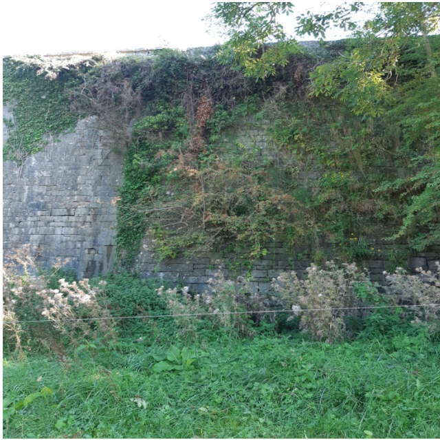
Albert Bridge Clonmel – Before works
