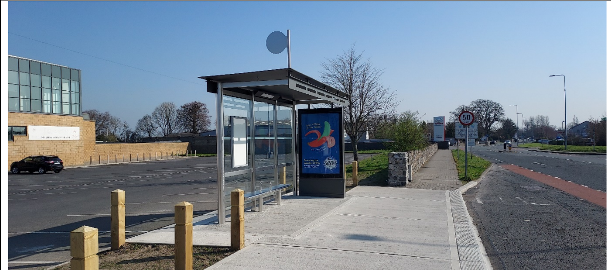
Bus Shelters recently completed at Springfort Retail Park, Nenagh – Northbound
