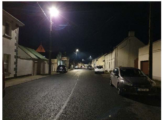
Drangan After Lighting Upgrade
