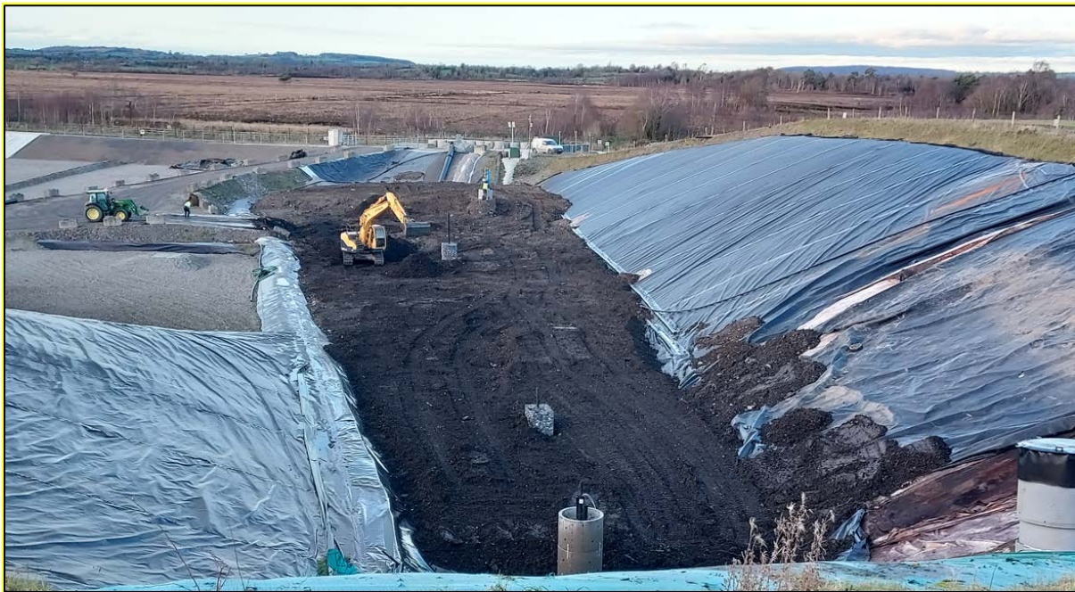
Ballaghveny Landfill – Filling of the Wedge Cell
