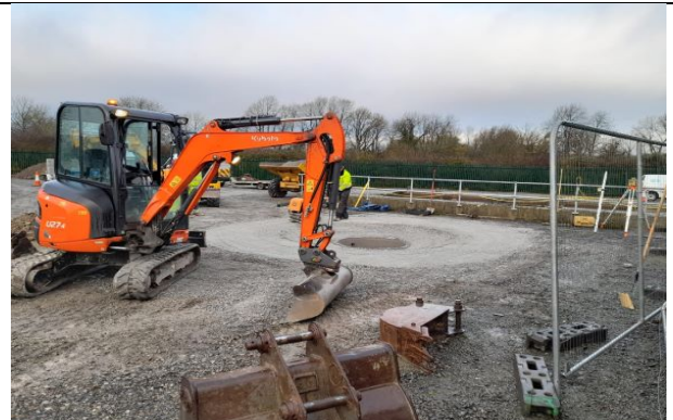
Upgrade Works at Borrisokane Wastewater Treatment Plant
