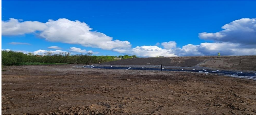
Tipperary Town Landfill Remediation Project – Preparation for installing the LLDPE Liner
