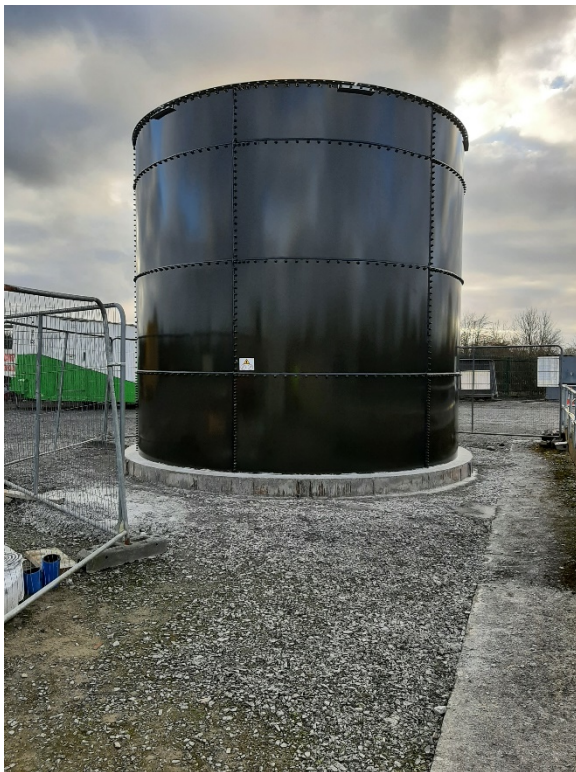
Borrisokane WWTP Upgrade Works
