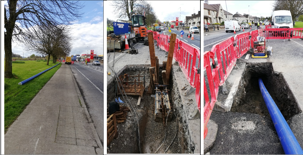
Watermain Rehabilitation Carrick-On-Suir
