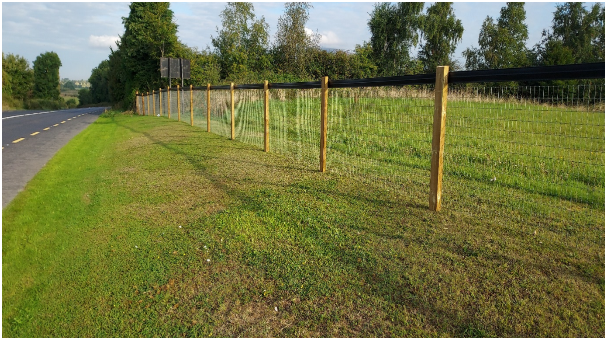
Retrofit fencing on N24 Carrick on Suir MD
