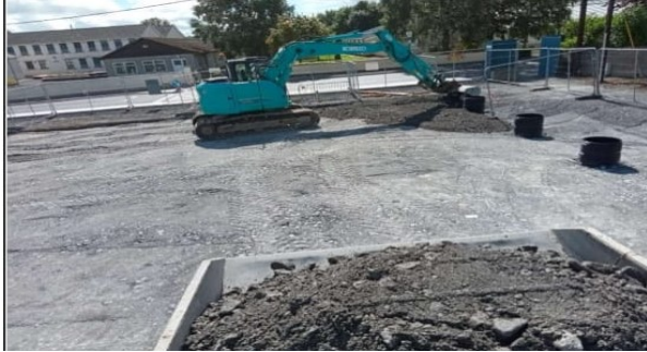
Works on Car Park
