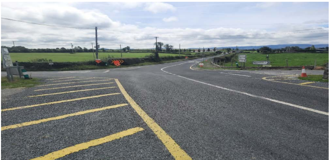
R493 Knigh Cross Improvement Works
