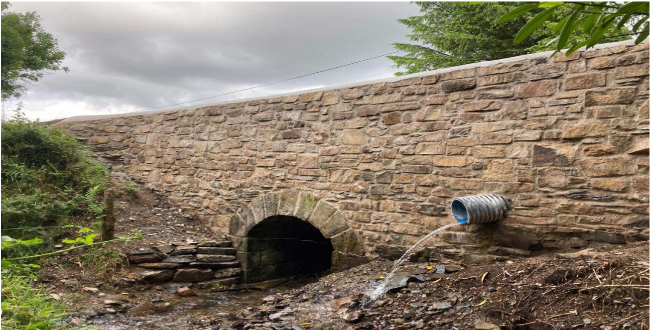
Bridge repair works at Shanballyedmond, Rearcross – Summer 2022
