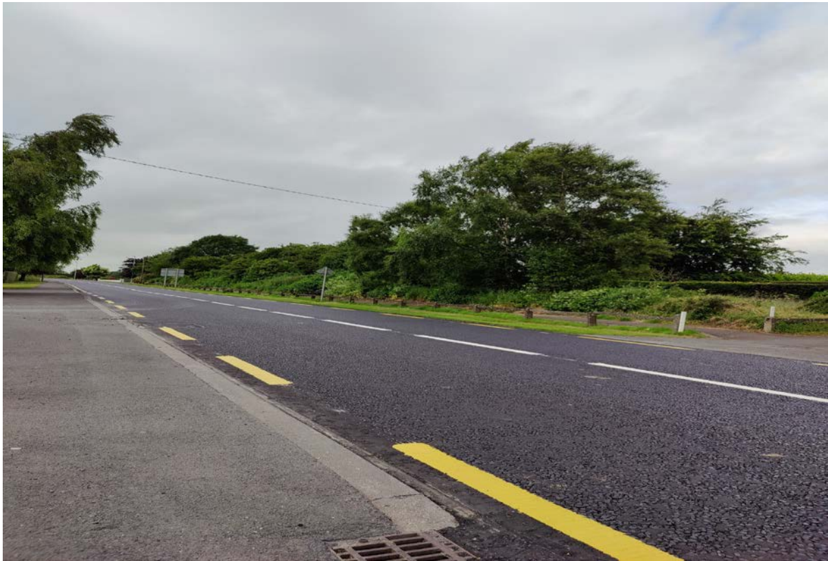
Capital Maintenance Works – N62 Brittas Road, Thurles
