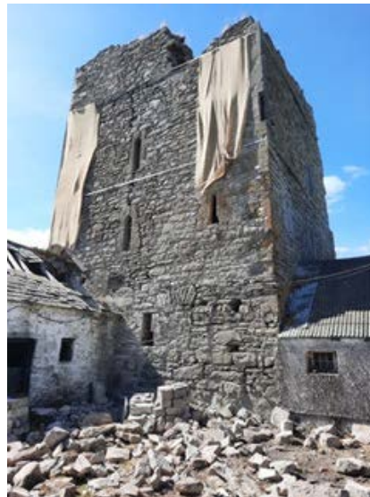
Completed works at Coolquill Castle and Boolabaun Castle for 2022.
