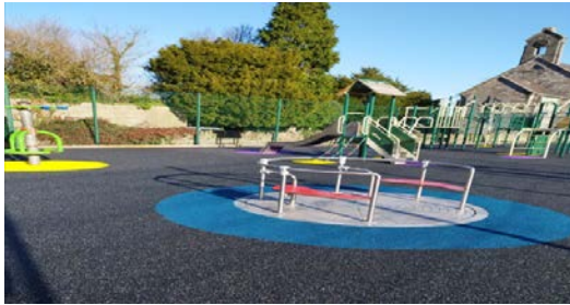
Upgrade of Clogheen Playground delivered by Tipperary-Cahir-Cashel MD – Clár funded
