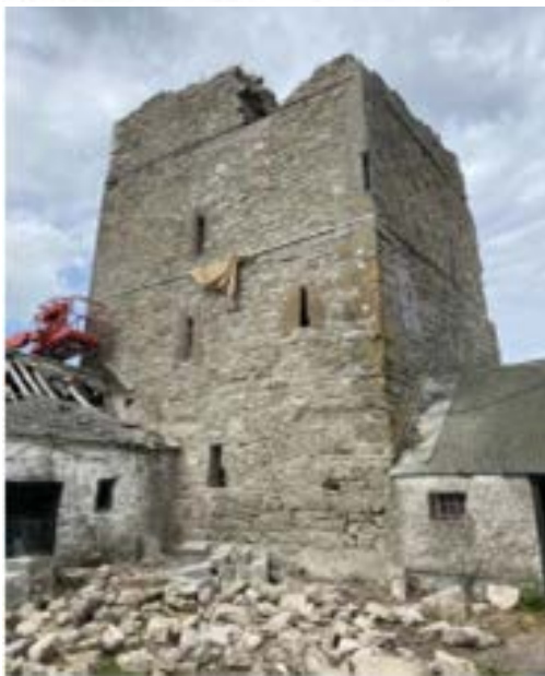
Before and after photos of works at Boolabaun Castle
