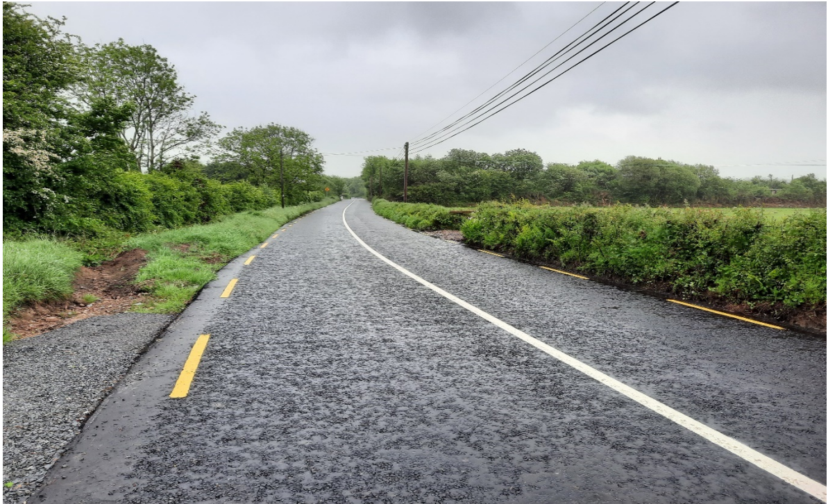
Restoration Improvements Works - R503 Rosmult
