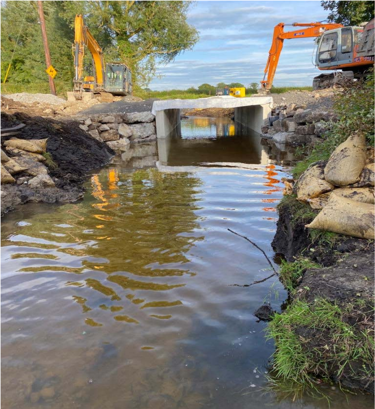
Bridge Rehabilitation Works at Kilclonagh, Moyne
