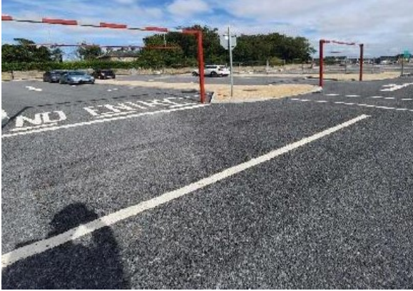
Works on Car Park
