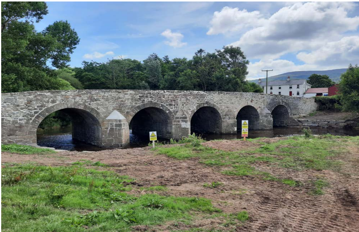
Cappa Old Bridge Remedial Works
