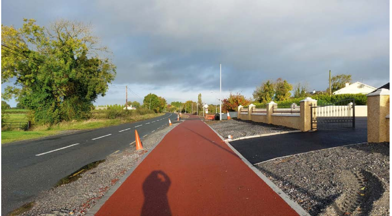
Riverstown Shared Surface - Active Travel project
