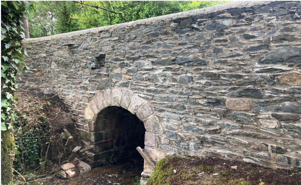
Bridge Rehabilitation Works - Shanballyedmond Bridge, Rearcross
