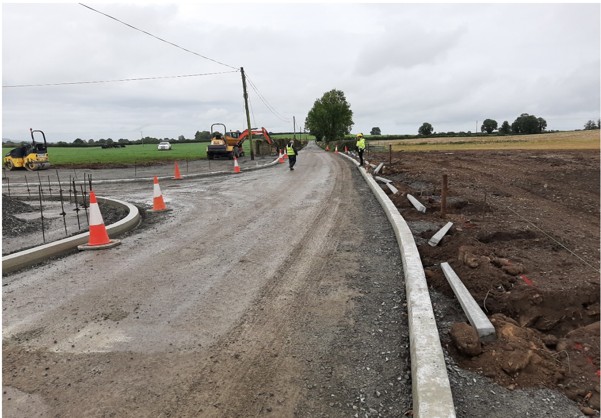
Safety Improvement Works – Road Realignment L3211, Roadstown Road Junction
