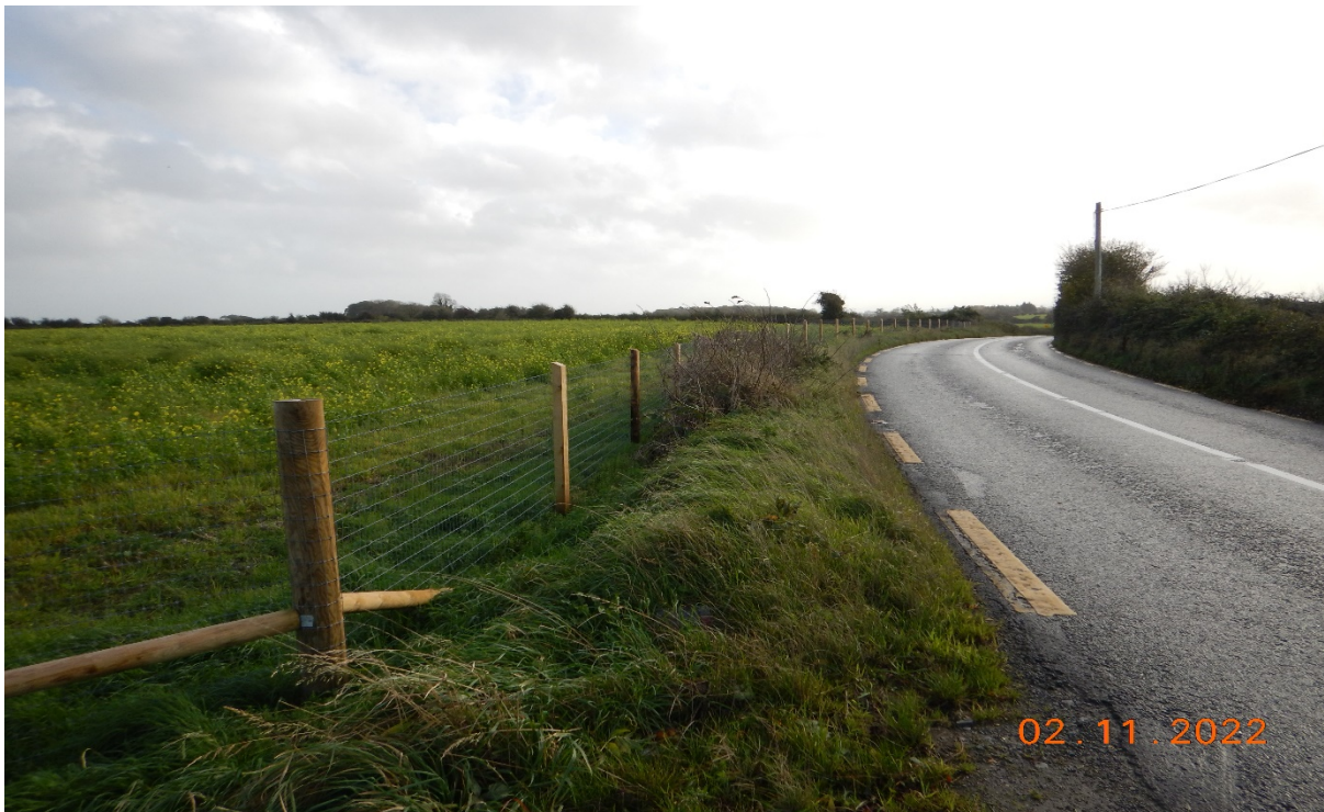
Retrofit fencing on N65 at Ballyspillane, Borrisokane
