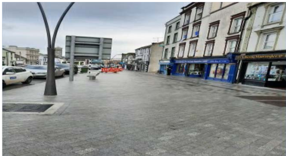
Liberty Square Phase 1 Completed
