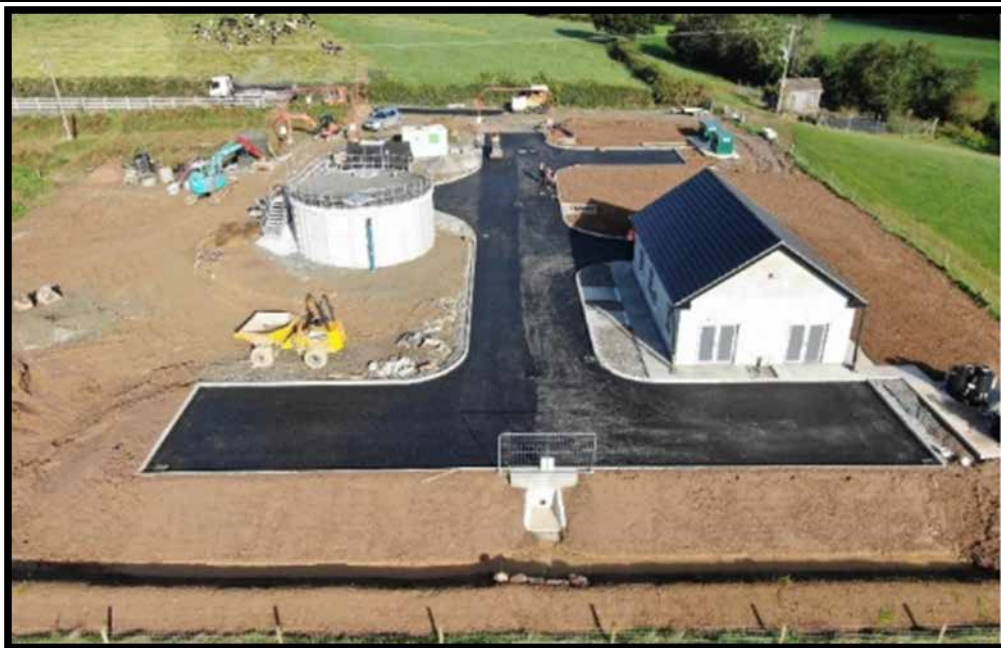
Photograph No. 1: Ardfinnan Regional Water Supply Scheme water treatment plant at Scart East, Ballylooby, Cahir.
