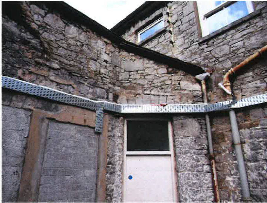
East Inner Yard Looking West
