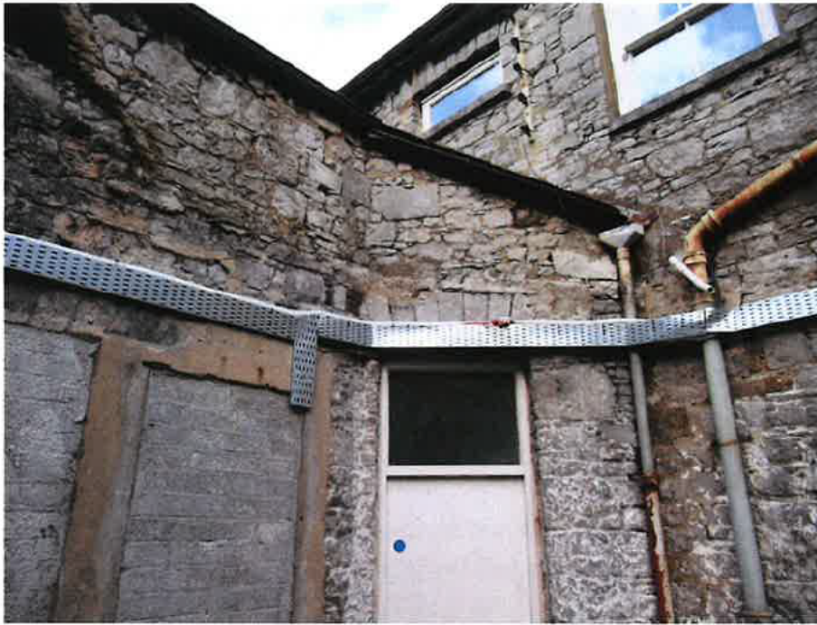
East Inner Yard Looking West
