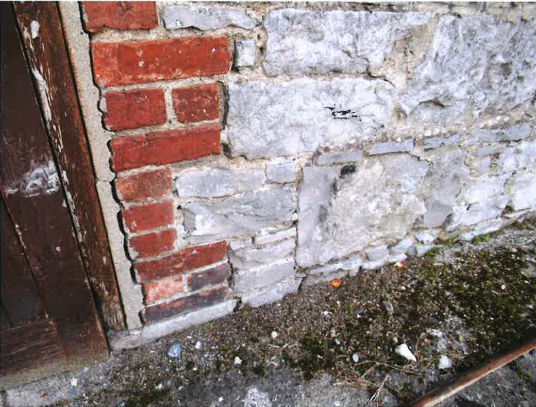
Former Hall West Side
