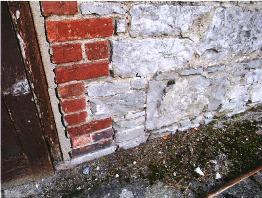
Former Hall West Side
