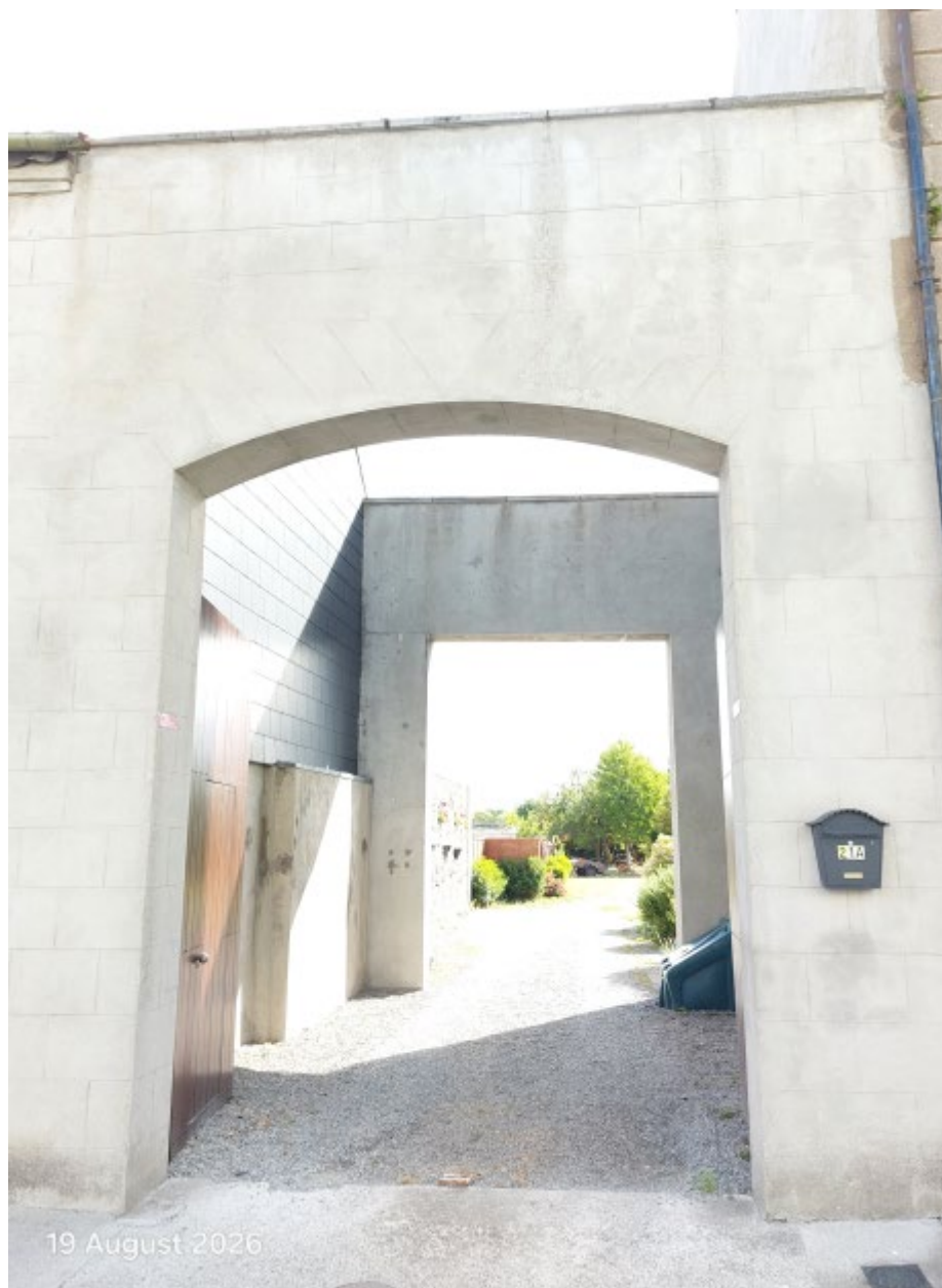
Figure 1 Entrance onto New Street
