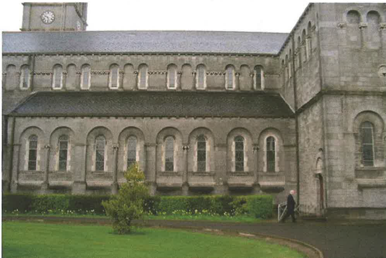
Fig. 4: East façade of the Cathedral of the Assumption showing replacement fibre cement slates to the high-level roof (of the nave) and lean-to roof of the side aisle.
