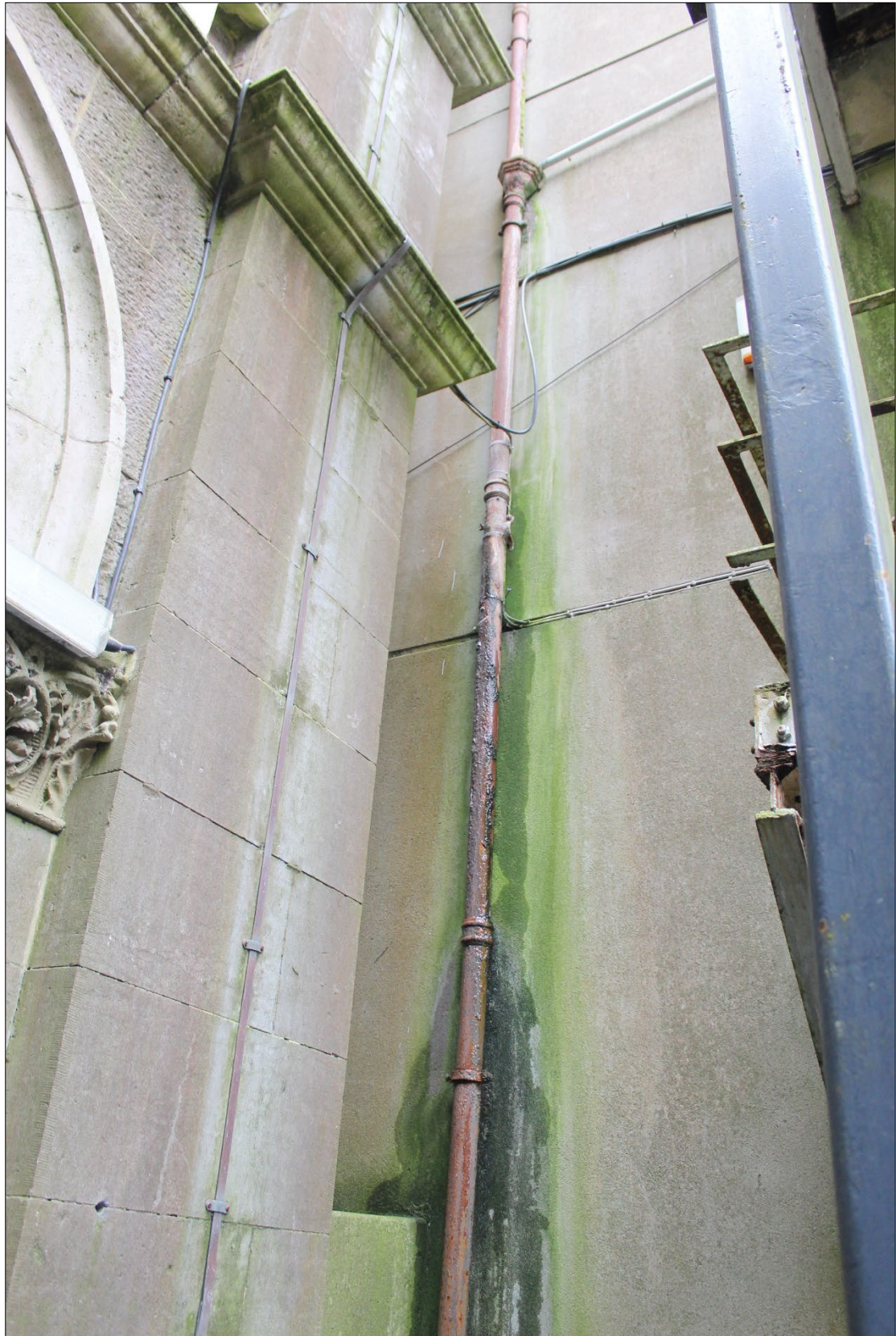
Figure 6: Existing historic cast-iron rainwater goods should be retained and repaired where possible with new cast-iron rainwater goods referencing historic detail surviving on site or visible on historic photographs. All downpipes should be fitted to facilitate access for inspection, maintenance and painting. All hoppers should be fitted with overflow pipes to give the earliest possible warning to building management staff of stormwater blockages at high level.
