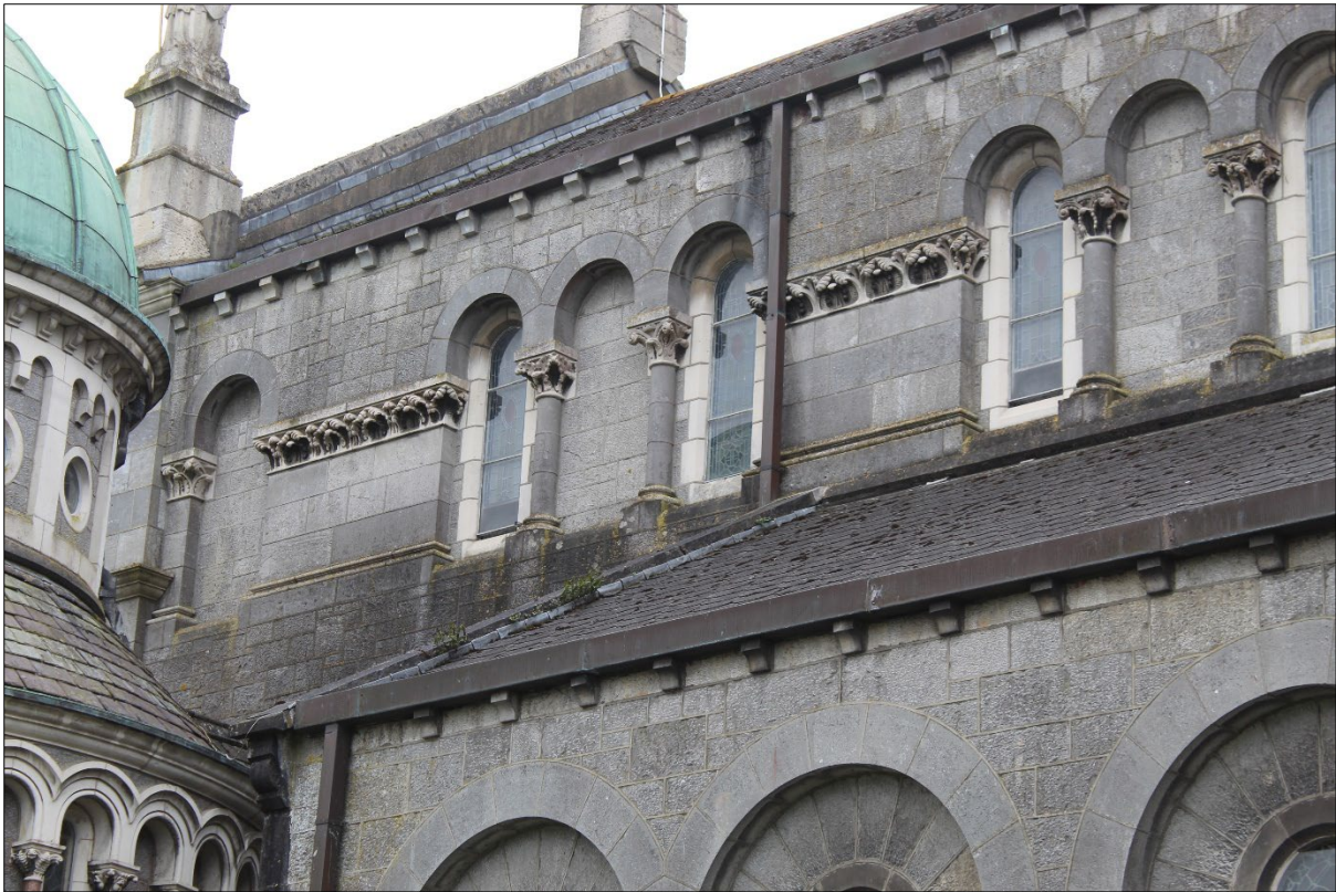
Figure 3: Roof of east aisle and southern part of east side of nave roof.
