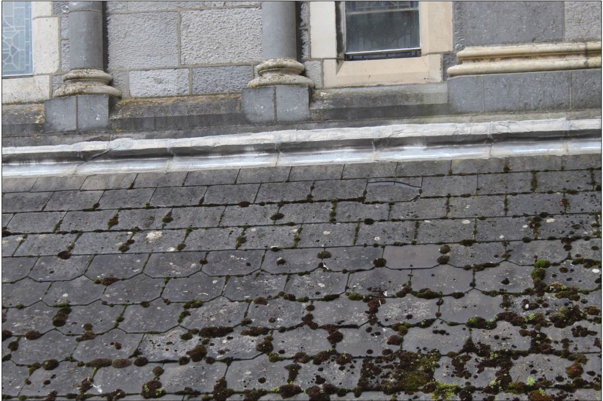
Figure 5: Abutment between roof of aisle and west elevation of nave
