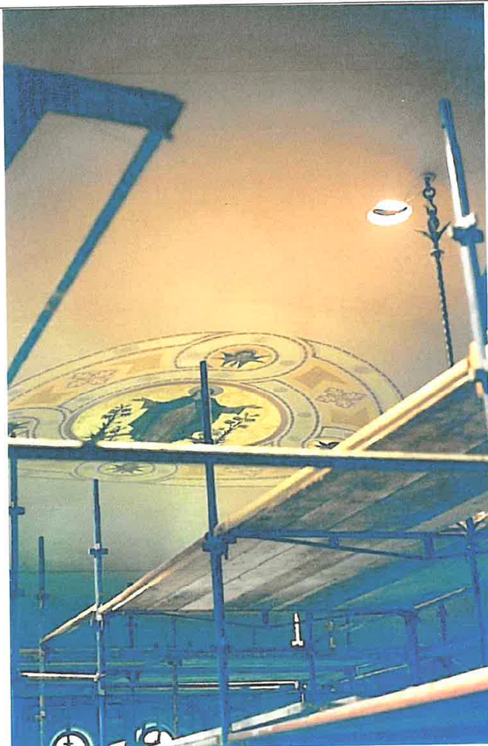
Historic decoration on sanctuary ceiling, prior to conservation and restoration (2002)
