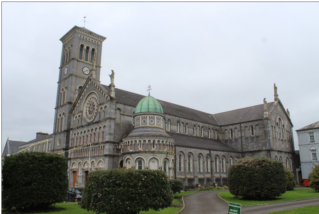
Figure 1: South façade and east side elevation of Cathedral of the Assumption, Thurles. Exact extent of replacement of existing polished granite columns with reinstated polished red sandstone on proposal drawings is required.
