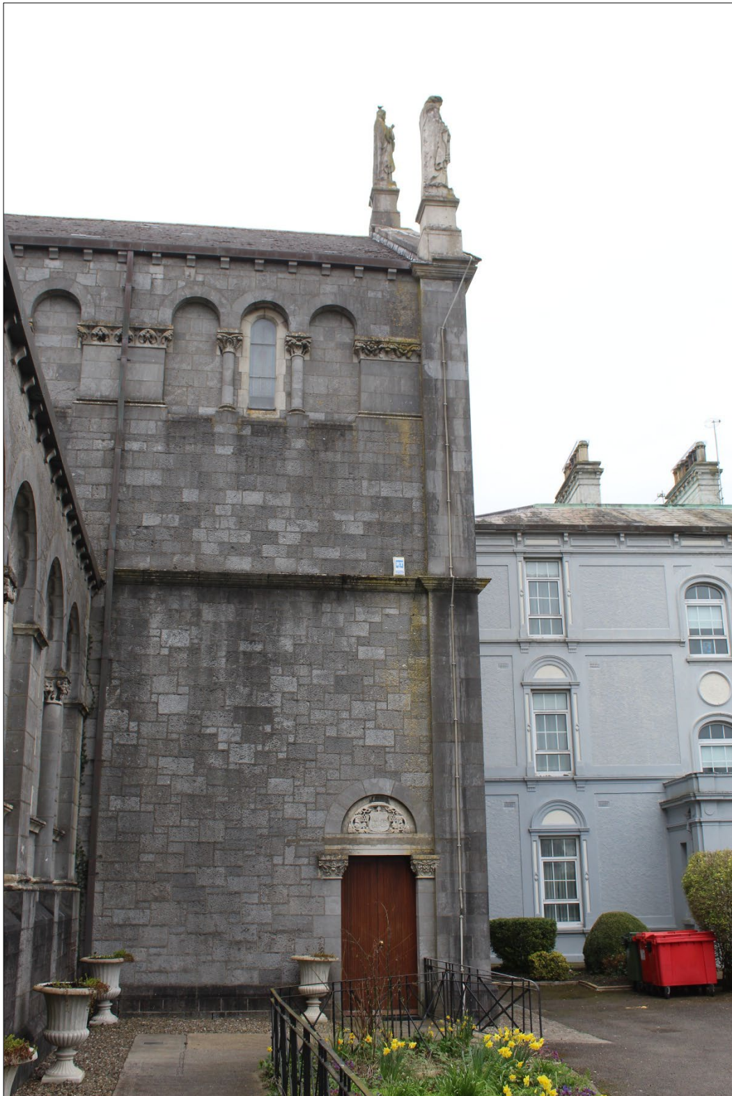
Figure 2: South elevation of east transept.
